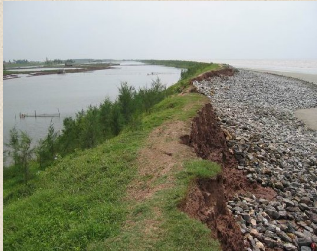
Sea dyke after the typhoon attack
