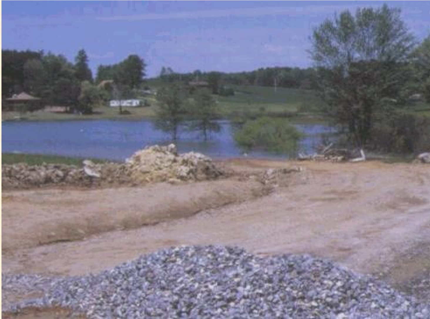
Illegal boat dock construction, Lake Chatuga, Georgia (USA)
