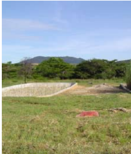
Example of a constructed wetland treatment system
