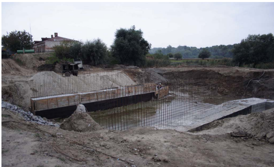
Fig. 3. Ongoing restoration works
