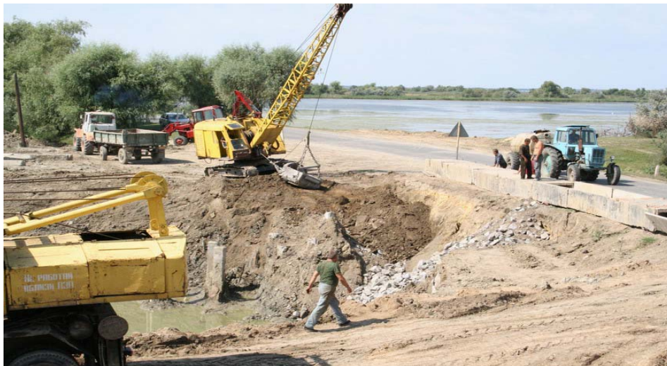
Fig. 2. Start of restoration works: construction of opening to the Danube with a bridge
