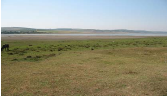
Figure 3. Upper part of the Cangaz water reservoir
