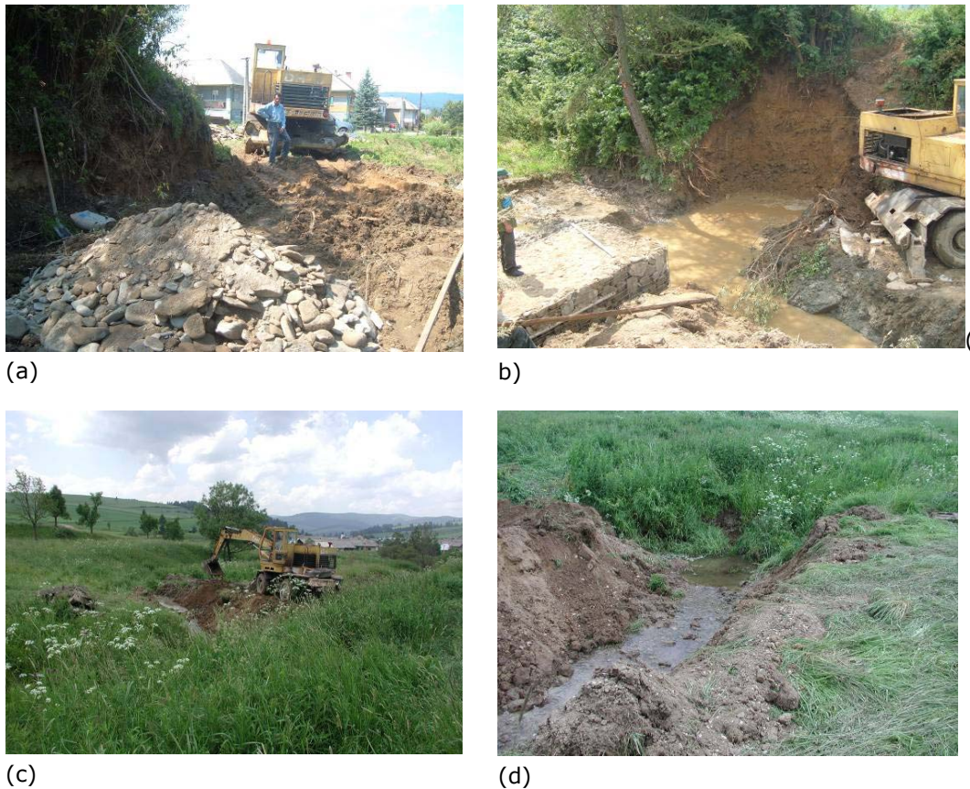
Figure 8: Technical implementation of measures to improve the situation of wetlands in the Slovakian pilot site – building small dams to control channel erosion (a,b) and re-opening of small meanders to improve ecological integrity of the canalized river and to lower discharge velocity (c,d).
