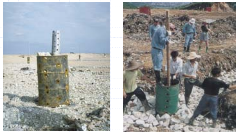
Gas Venting pipe using waste oil drum
