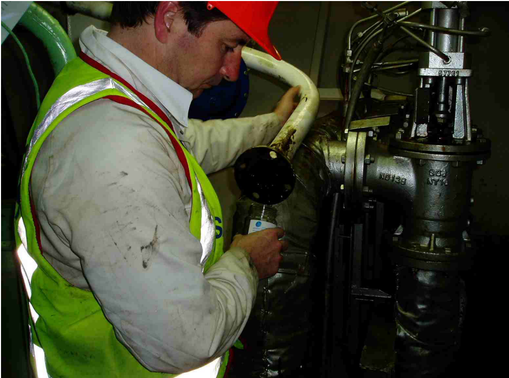
41. Samples being taken in the engine room.
