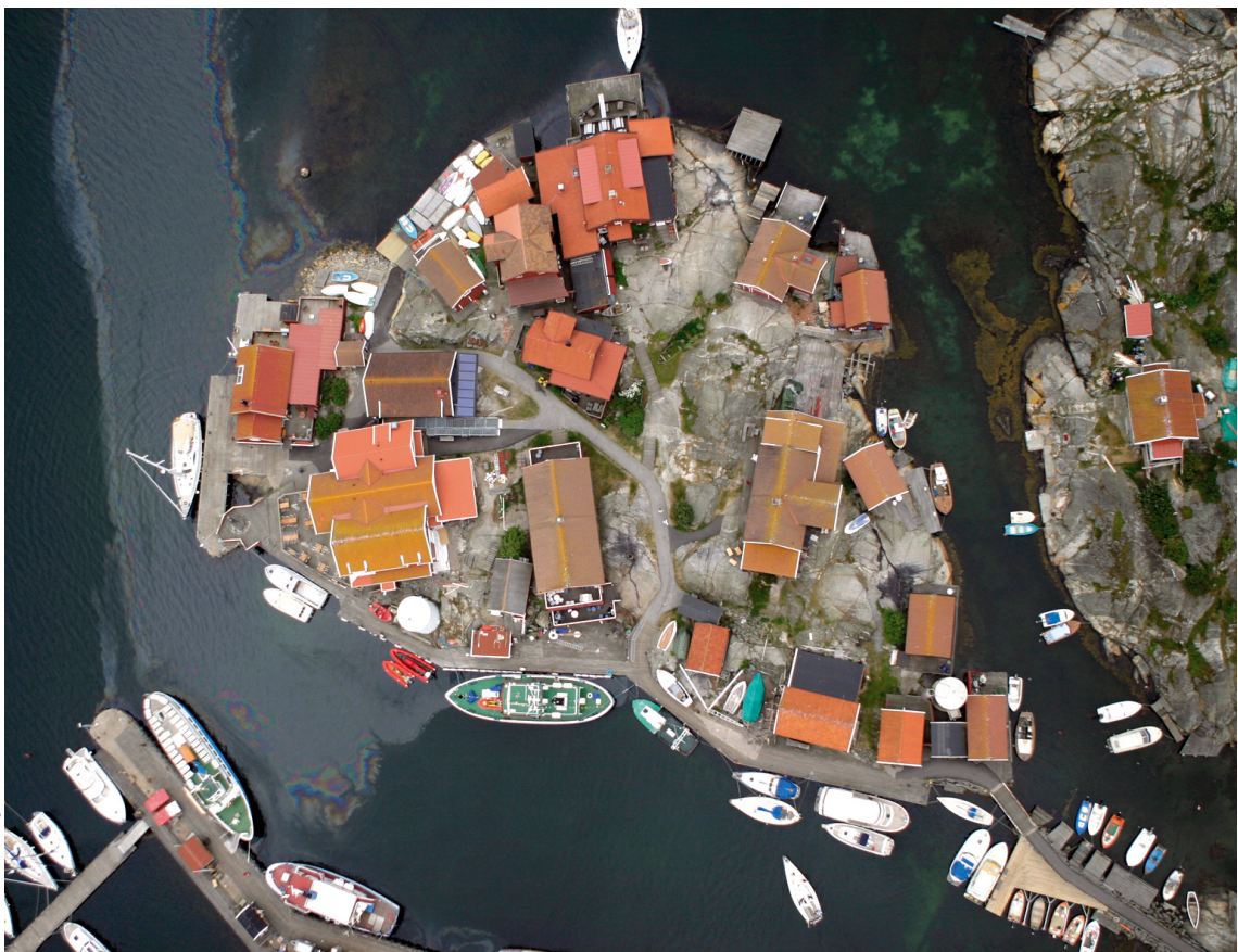
42. Property damage from oil discharge.
