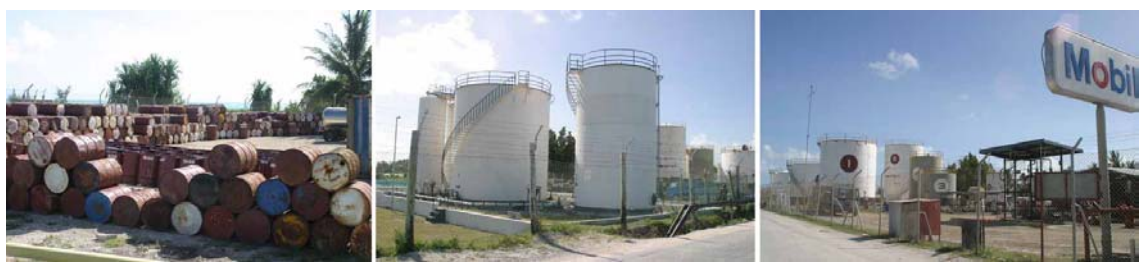
Figure 1-4 - KOIL Storage on Betio, Tarawa
