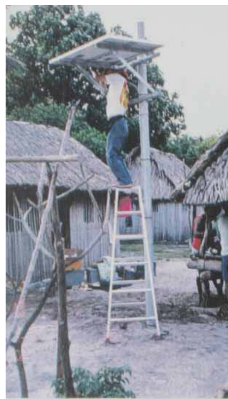
Figure 4-4 - Household panel Installation
