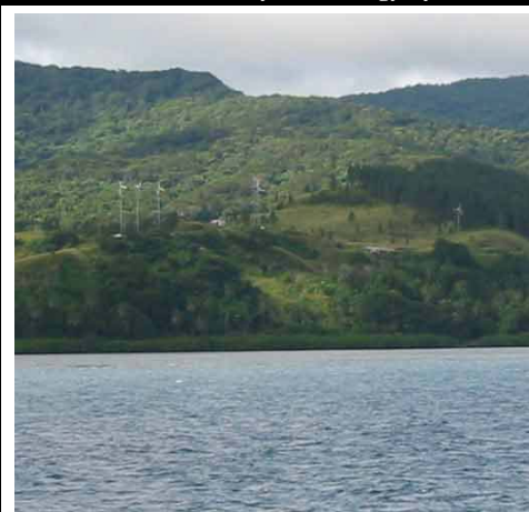
Figure 5-23 – The Nabouwalu Hybrid Energy System
