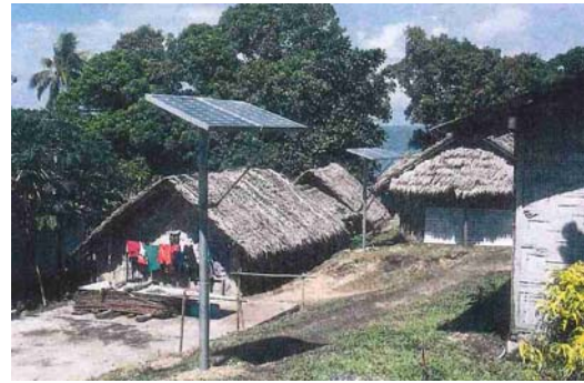
Figure 4-1 – JICA Solar PV Home System, Vanuatu
