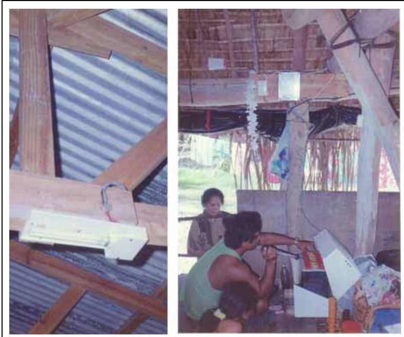
Figure 2-2 – Solar lighting systems in Tuvalu
