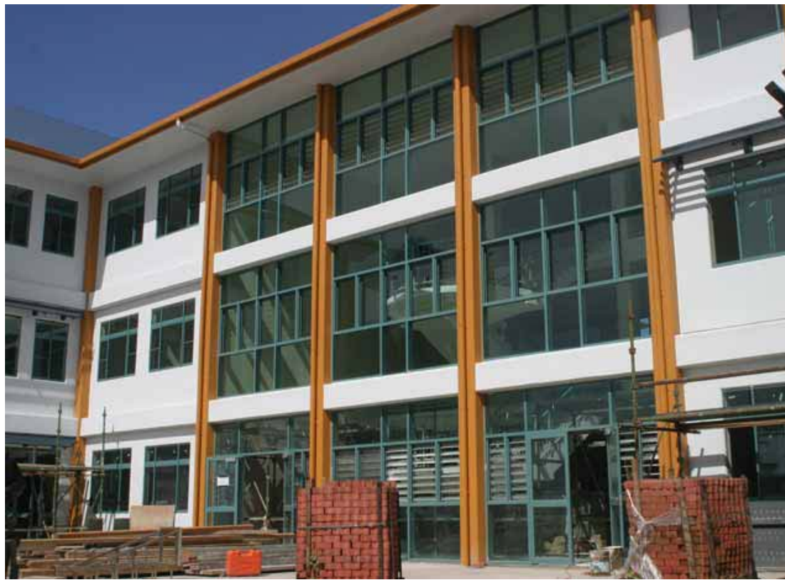
Figure 5-1 – New office building, west facing facade
