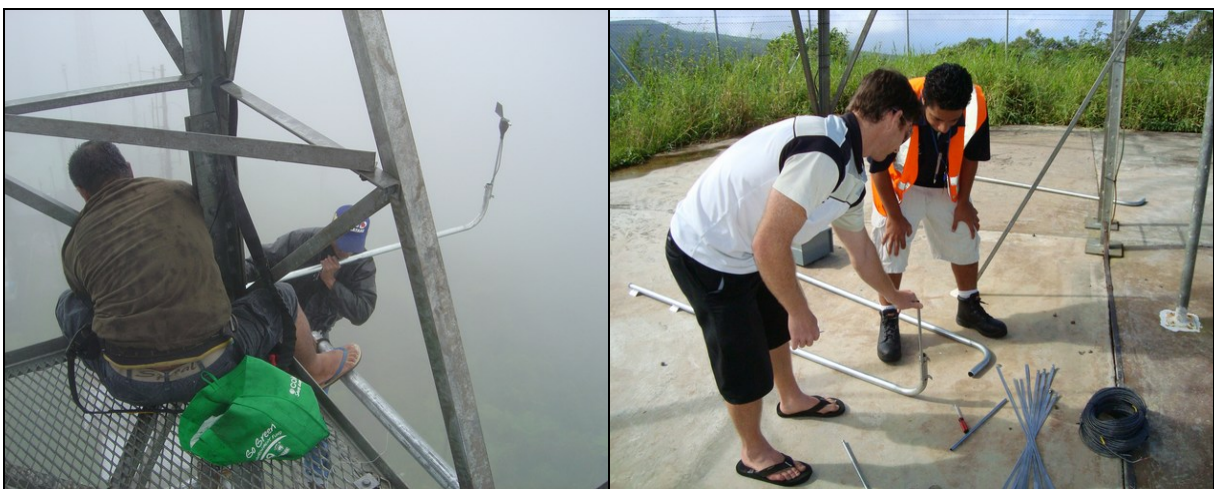
Fig 5: EPC staff members installing wind monitoring equipment on 34m telecommunication tower
