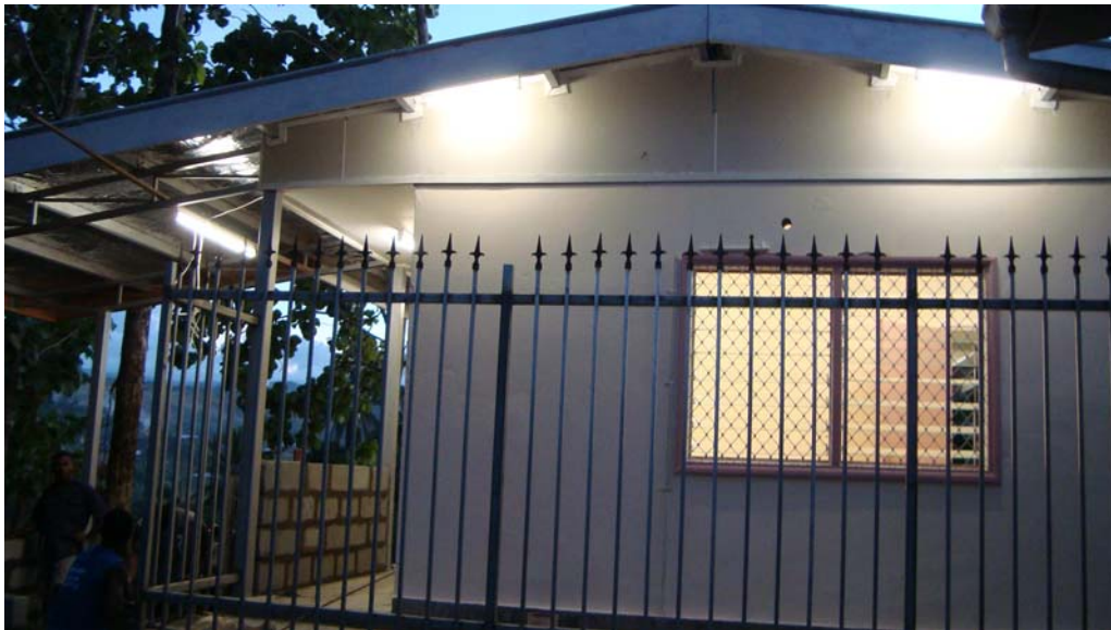
Fig 6: End view of the newly constructed RE Information Centre behind the Energy Office
