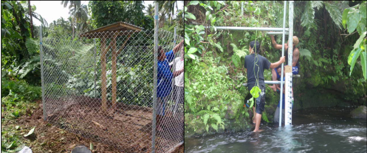
Fig 4: Construction of the Gauging station at Tafitoala.
