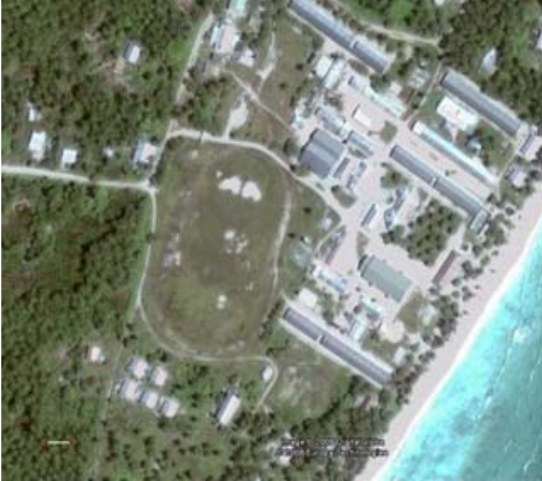
Fig 13: Aerial Photograph of Motufoua Secondary School
