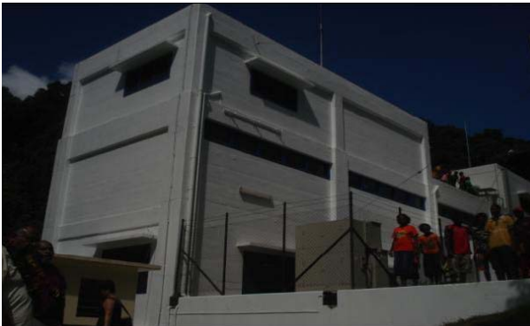
Fig 24: Sarakata Power station
