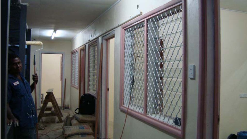
Fig 7: Along the corridor of the newly constructed RE Information Centre
