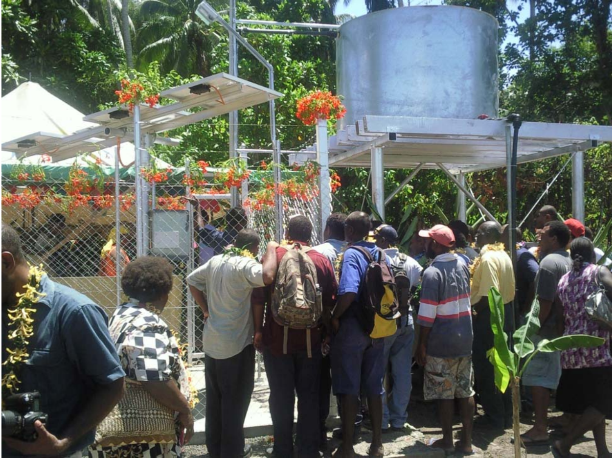
Figure 7: Commissioning of the California Village Solar PV (340 watts) powered water pumping
