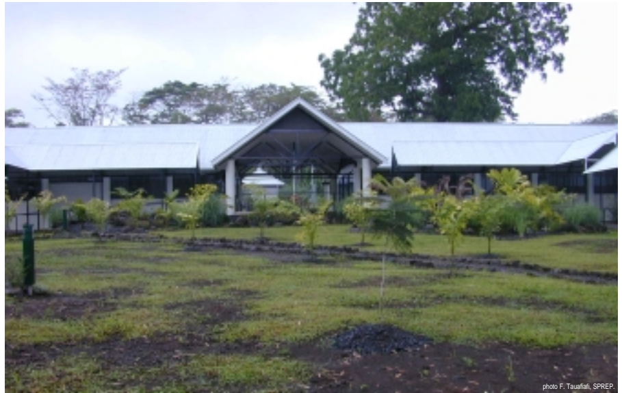
Rear view of the SPREP Centre complex
