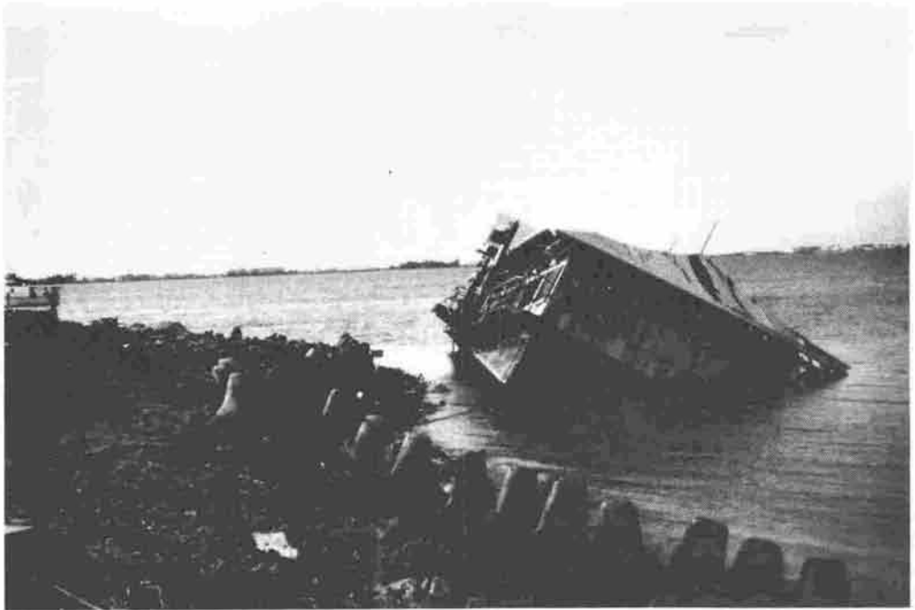
Plate 3: Uluga: Lagoon 'Sea Wall' and Storm Damaged Restaurant
