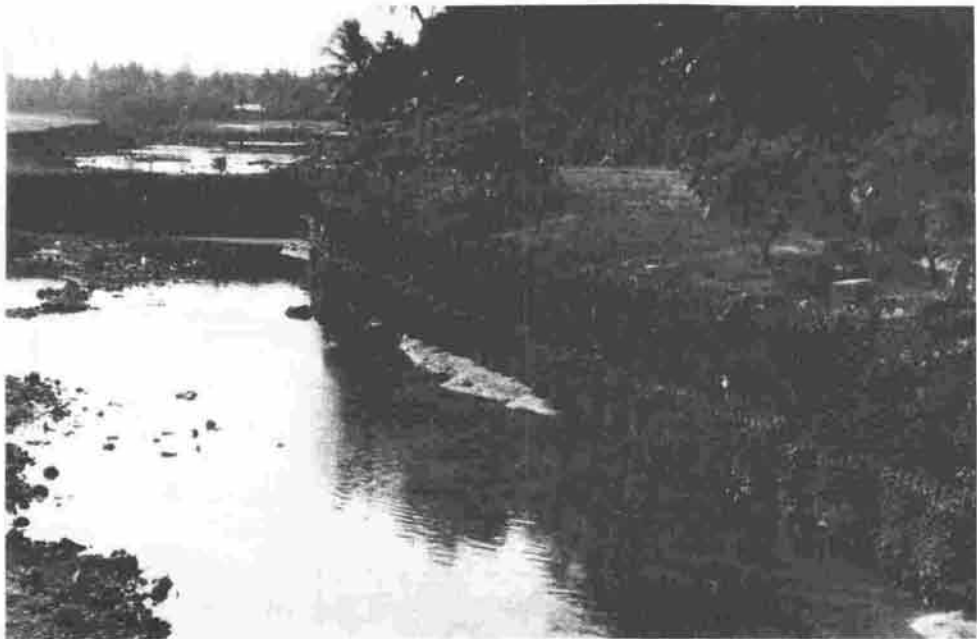
Plate 4: Rairok: Gabions on Seaward Coast
