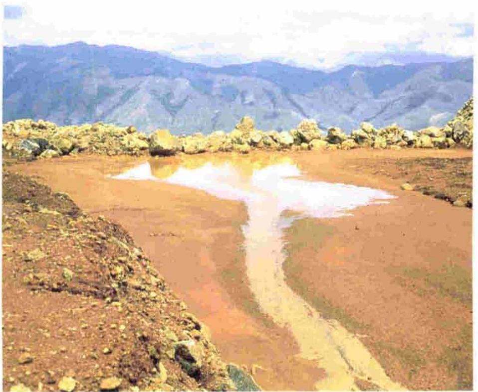
A protective dam of boulders traps the finer materials on a spoil-dump.
