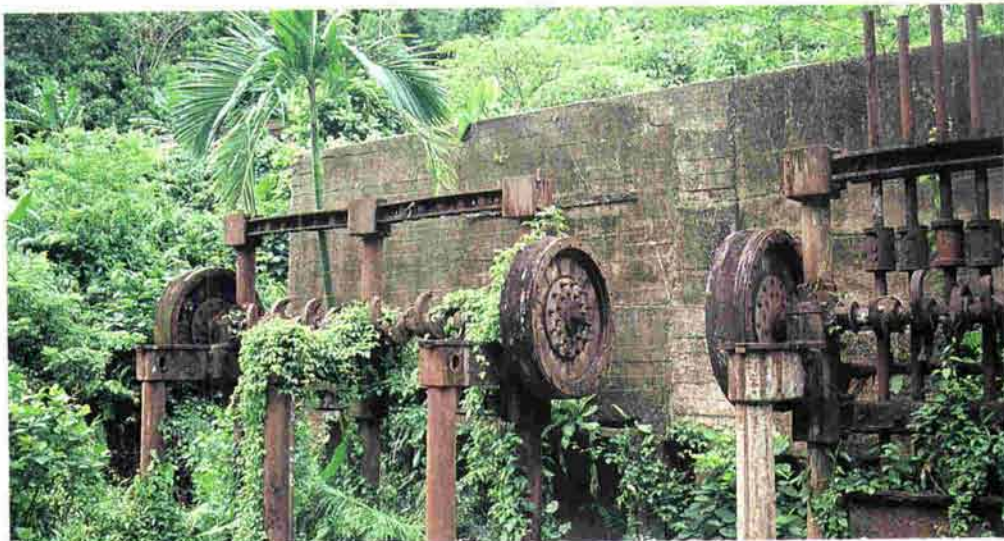
Derelict stamp battery used to crush the gold-bearing ore during the underground phase of mining.
