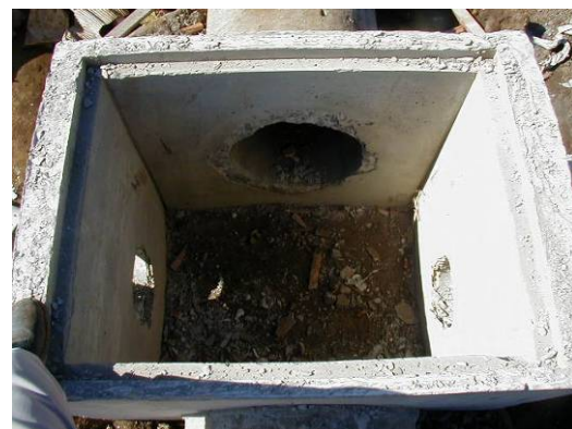
Photo- 24: Pipe Connection Pit
