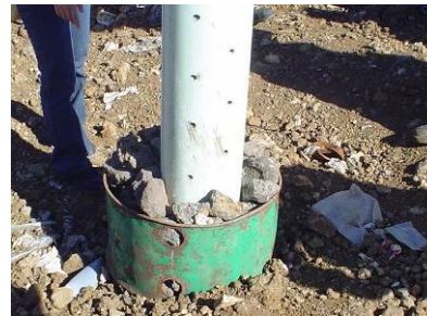
Photo- 27: Vertical Gas Venting Pipes at Landfilled Area
