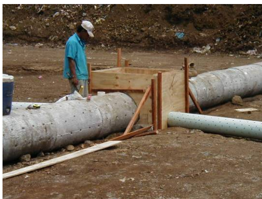
Photo- 24: Pipe Connection Pit
