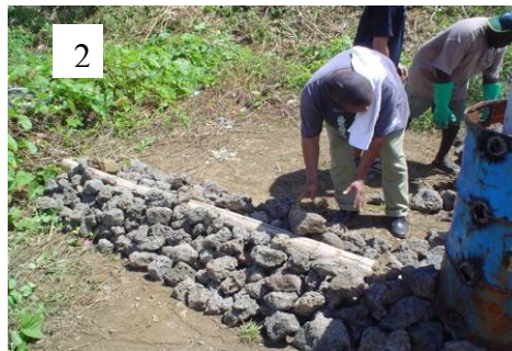
Photo- 27: Vertical Gas Venting Pipes at Landfilled Area
