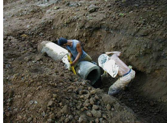
Photo- 15: Diversion Pipe Setting
