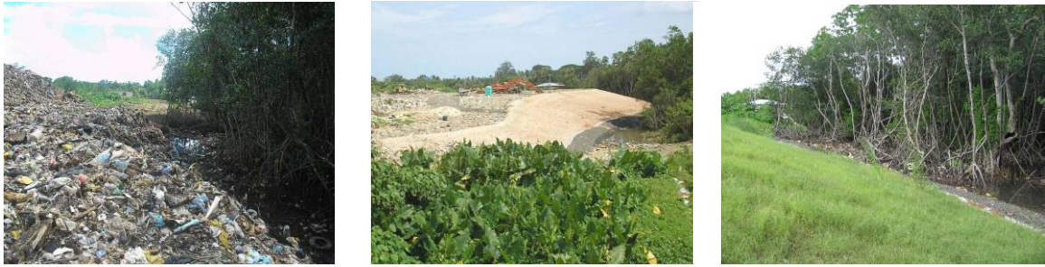
Photo- 41: Construction of Slope (M-dock Landfill, Palau)
