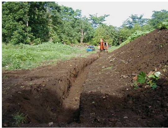
Photo- 13: Perimeter Drain Excavation
