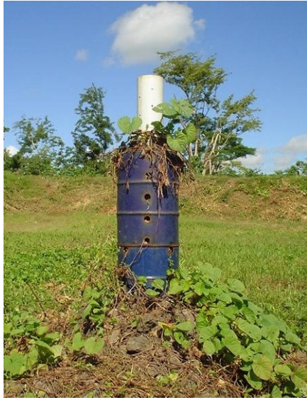
Photo- 27: Vertical Gas Venting Pipes at Landfilled Area
