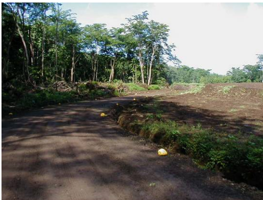
Photo- 11: Side Ditch with Curb Stone
