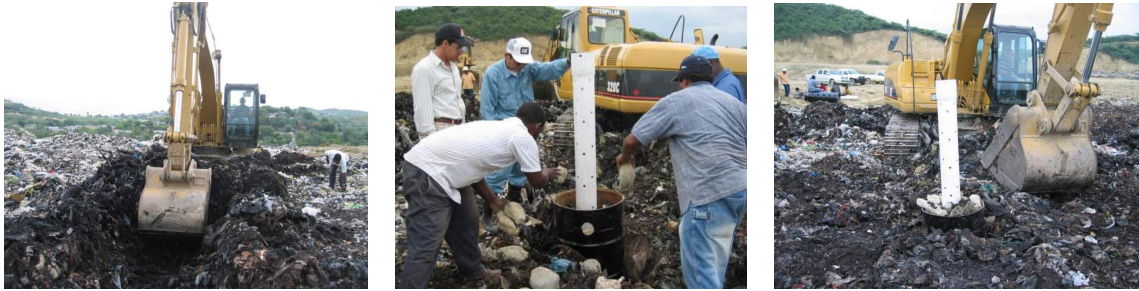
Photo- 47: Installation of additional independent gas venting facility
