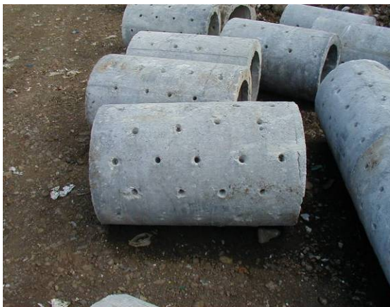
Photo- 17: Samples of Leachate Collection Pipe
