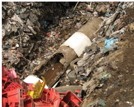
Photo- 42: Damaged Leachate Collection Pipes
