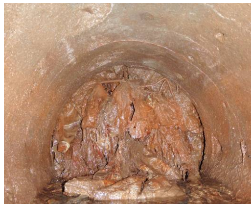
Photo- 43 Clogged Leachate Collection Pipes
