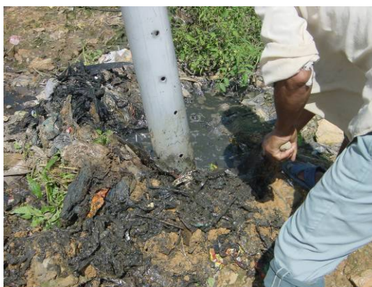
Photo- 44: Clogged Vertical Gas Venting Pipes
