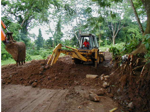
Photo- 14: Excavation of Trench
