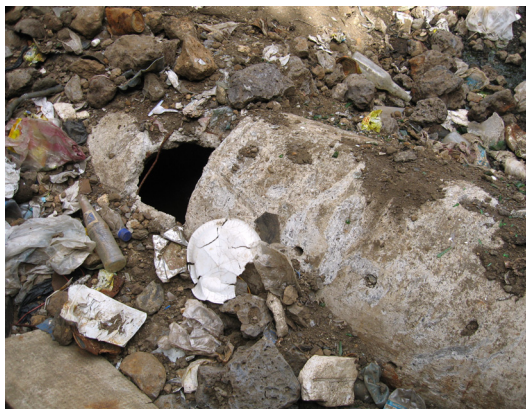
Photo- 42: Damaged Leachate Collection Pipes
