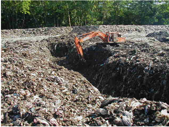
Photo- 21: Excavation of Trench at Deep Waste Layer
