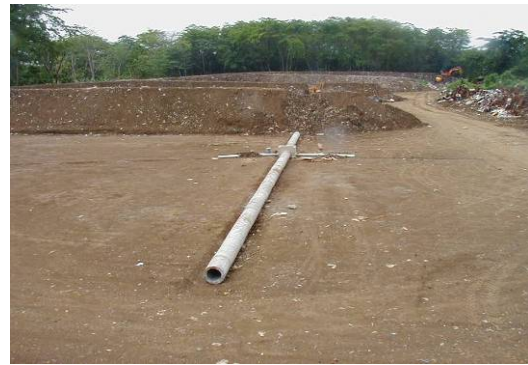
Photo- 19: Concrete Pipe Setting
