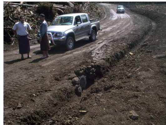
Photo- 12: Side Ditch with Road Crossing Culvert
