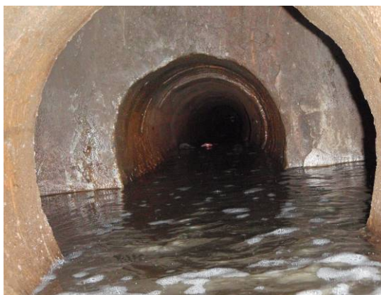
Photo- 43 Clogged Leachate Collection Pipes
