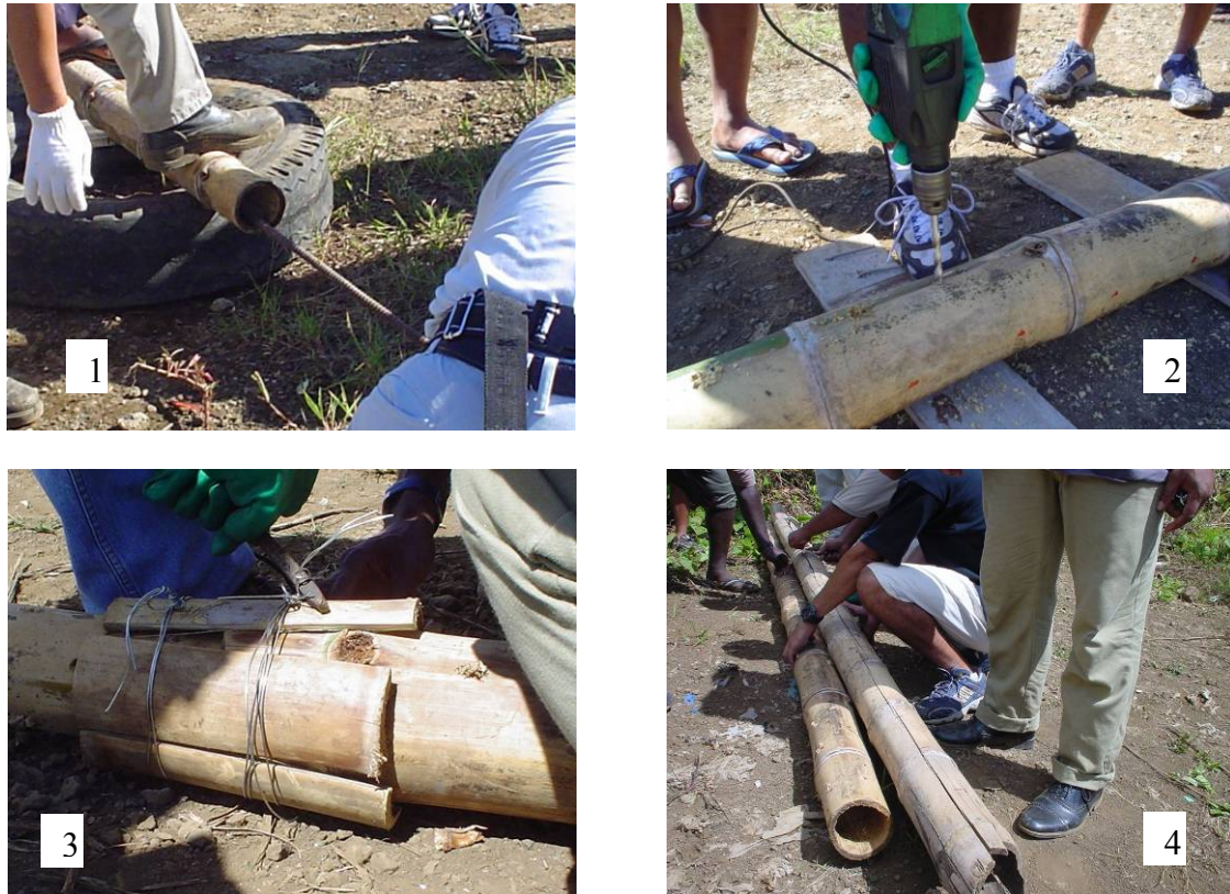
Photo- 18: Bamboos as Substitute Material for Pipes
