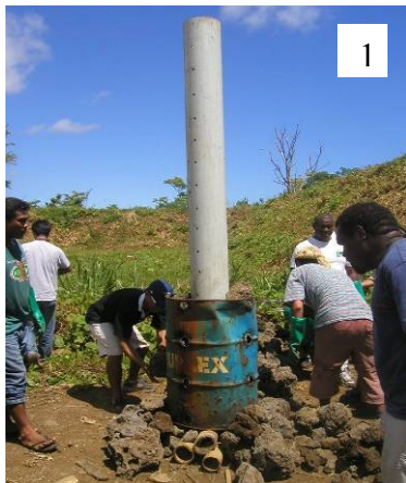
Photo- 27: Vertical Gas Venting Pipes at Landfilled Area
