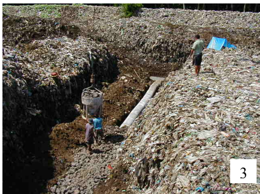
Photo- 22: Installation of Leachate Collection Facility in Deep Waste Layer
