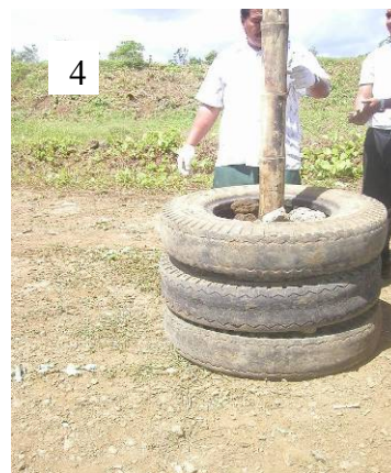
Photo- 28: Application of Used Materials for Leachate/Gas Control Facility
