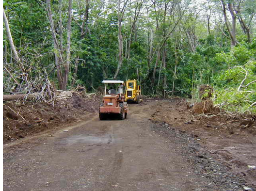
Photo- 9: Compaction & Gravel Paving
