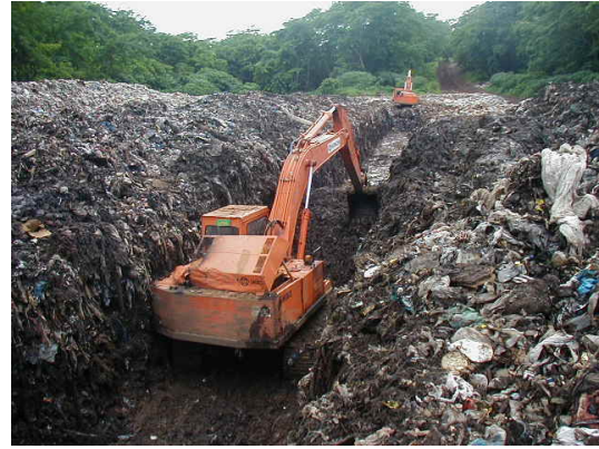
Photo- 21: Excavation of Trench at Deep Waste Layer
