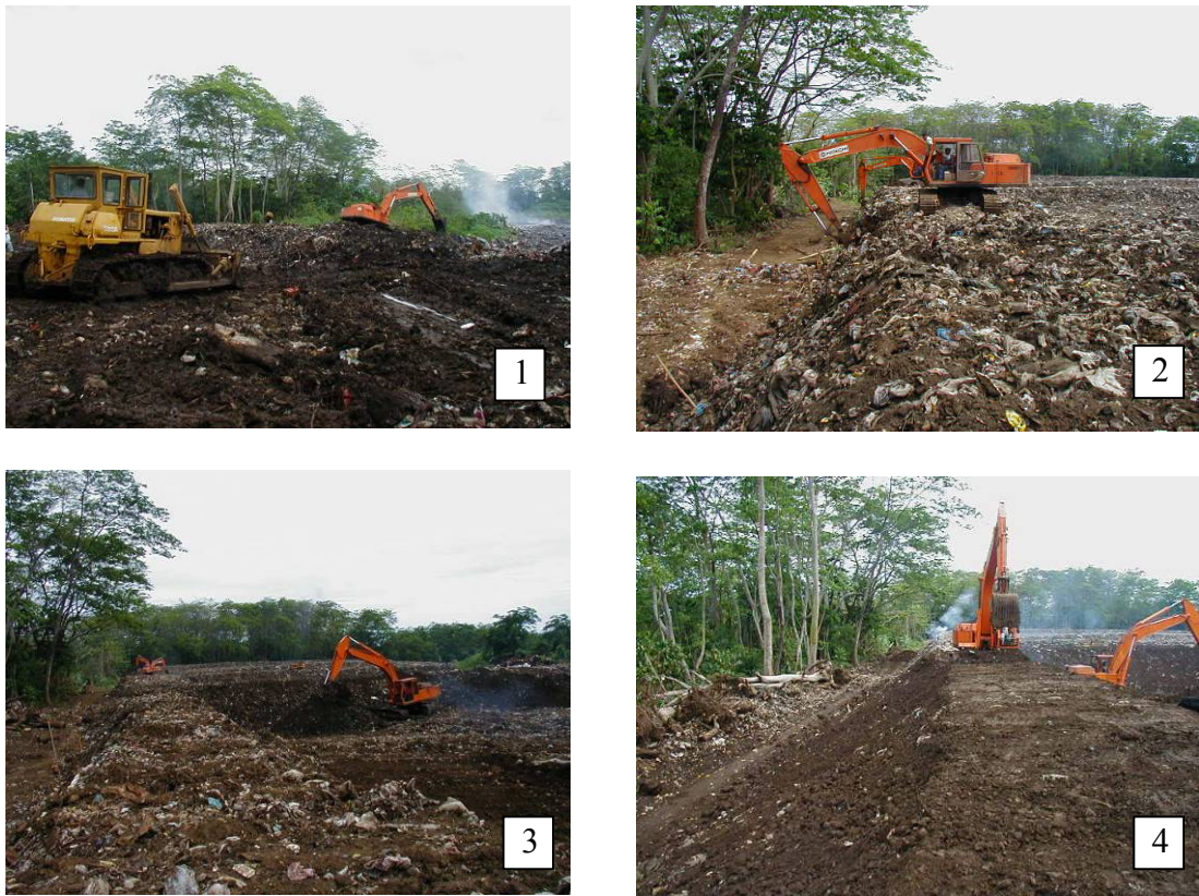
Photo- 16: Sequence of Enclosing Bunds Construction
