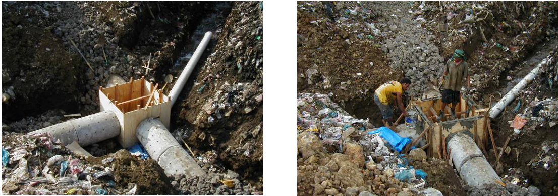
Photo- 25: Installation (in-situ concrete) of Connection Pit in Deep Waste Layer
