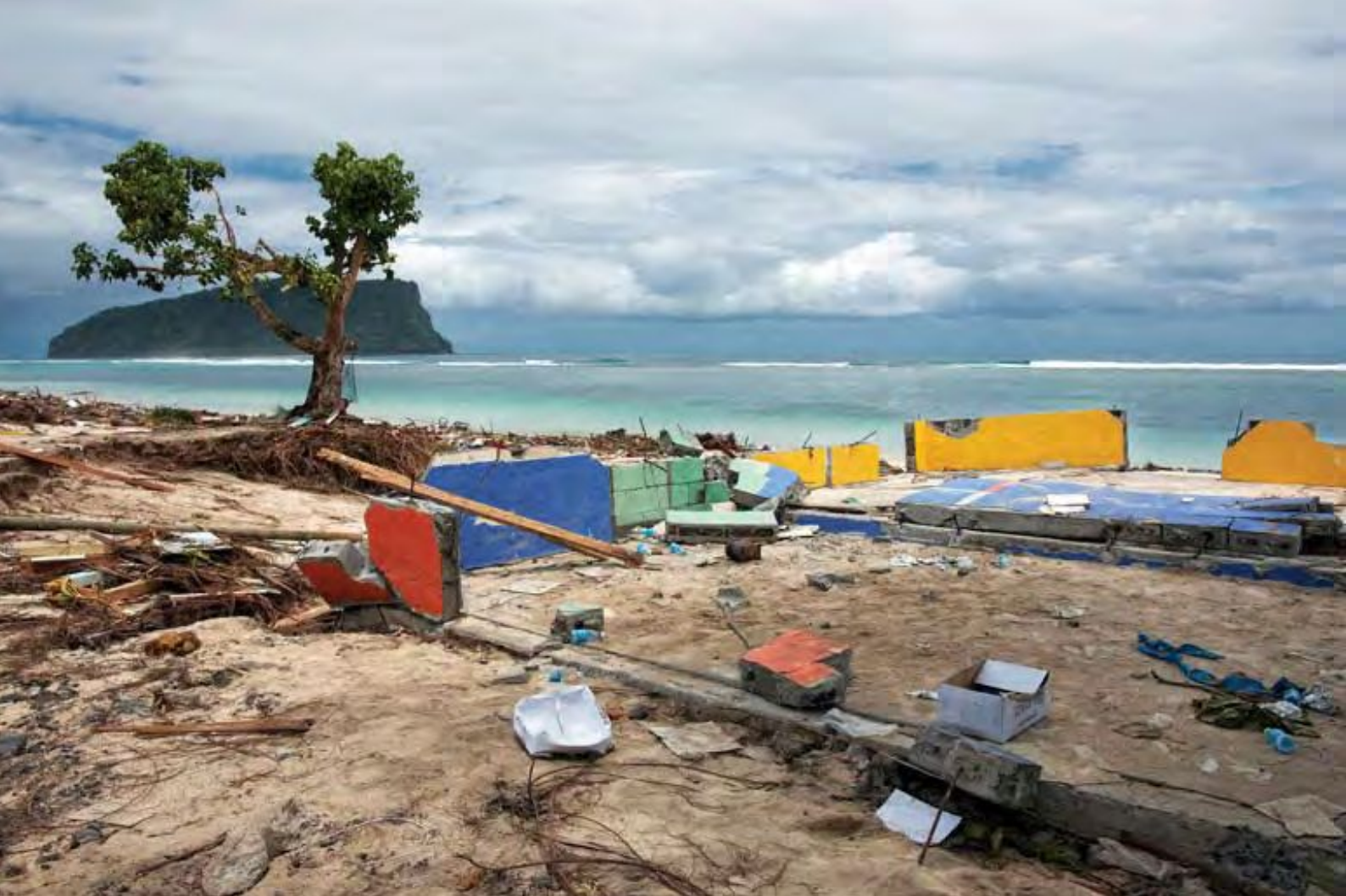
Shoreline destruction from 2009 tsunami at Lalomanu, Samoa PHOTO – STUART CHAPE
