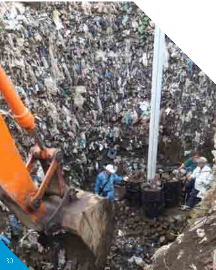
Tafaigata Landfill Rehabilitation Project in Samoa: Installation of semi-aerobic landfill aeration pipes.
