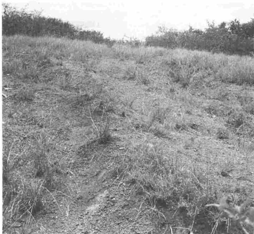
PLATE 4: Soil erosion is common in many Pacific island countries, often resulting from clearing land for forestry, road building or other activities. Careful use of EIA can reduce such occurrences markedly.
