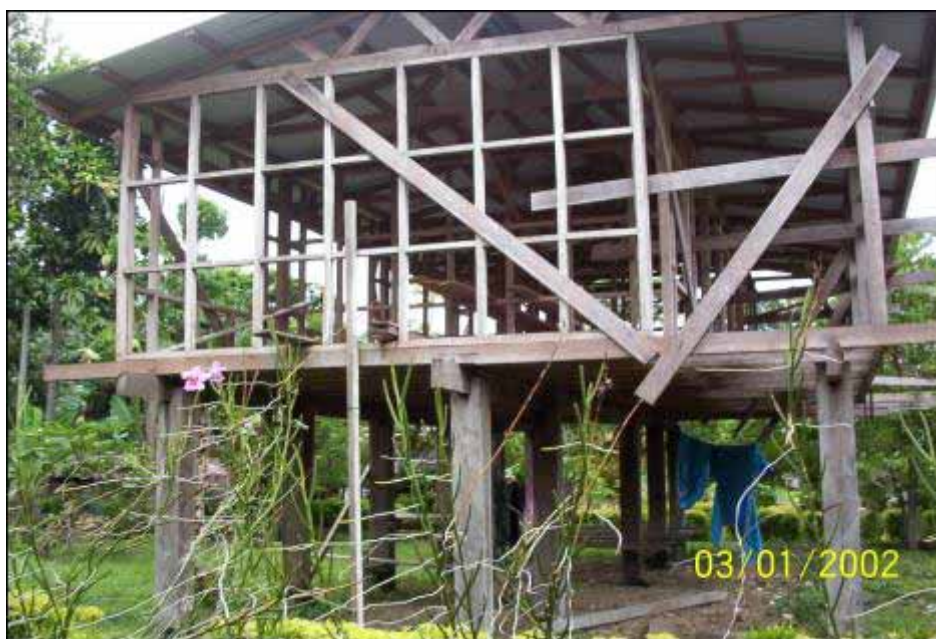
Plate 7: Guesthouse under construction at Chea
