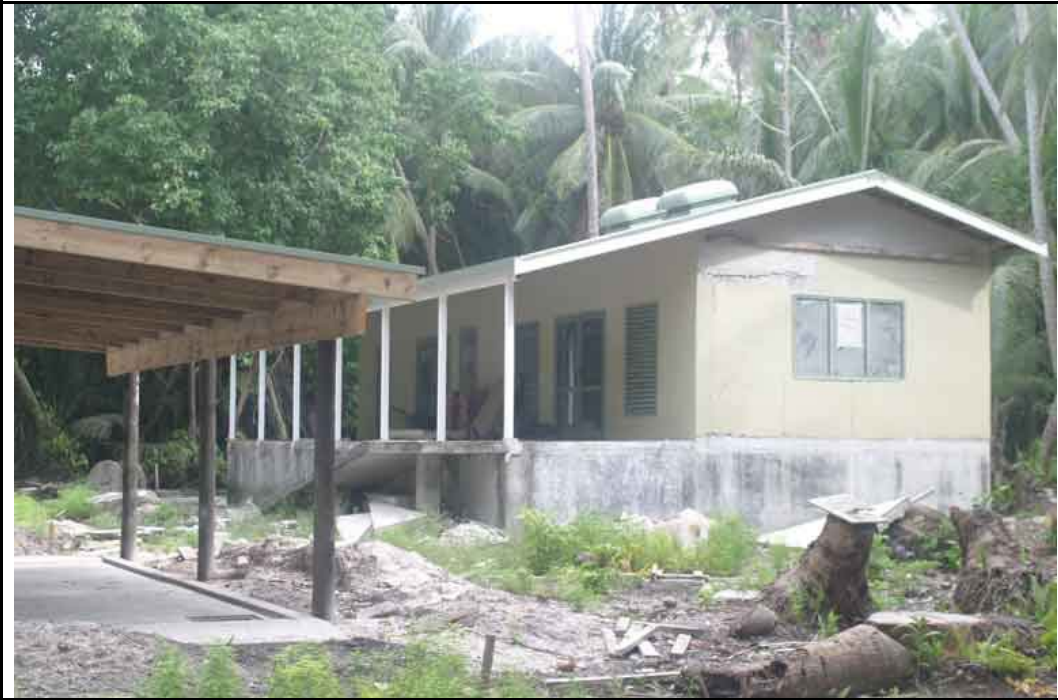
Figure 2-3 – New Power Station on Fakaofu
