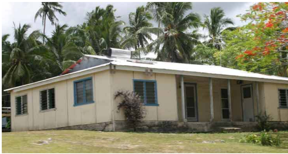
Home with solar water heating
