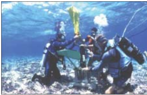
Figure 121 Divers installing a mooring buoy at Johnston Atoll (Photo: James Maragos).
