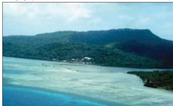
Figure 308. Causeway on Chuuk with remnants of a coral dredging operation from construction (Photo: James McVey).
