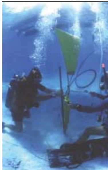
Figure 21. Installing mooring buoys at Johnston Atoll National Wildlife Refuge (Photo: James Maragos).
