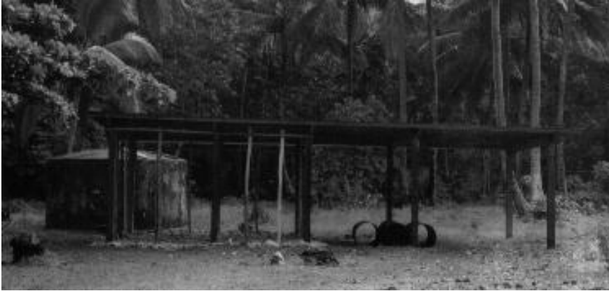
Fig: 9. One of three rainwater catchment and storage facilities
