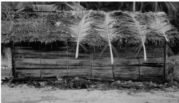
Fig: 5. Sleeping houses raised on foundation of rocks to accommodate flooding
