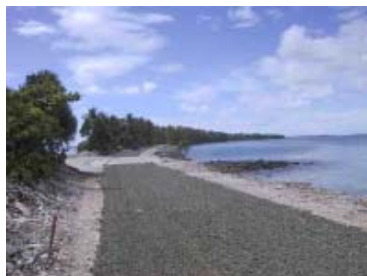
Upgraded road on Funafuti (photograph by Charles G. Kick, III, 2001)
