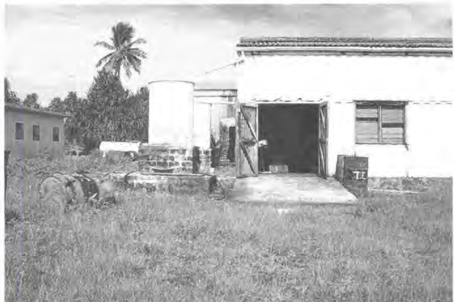
Back door of Funafuti Power Station. Oily wastes are simply hosed out the door, and drain away into the groundwater below. Managing oil waste is one of Tuvalu's most urgent pollution problems. (photo: Alefaia Semese)
