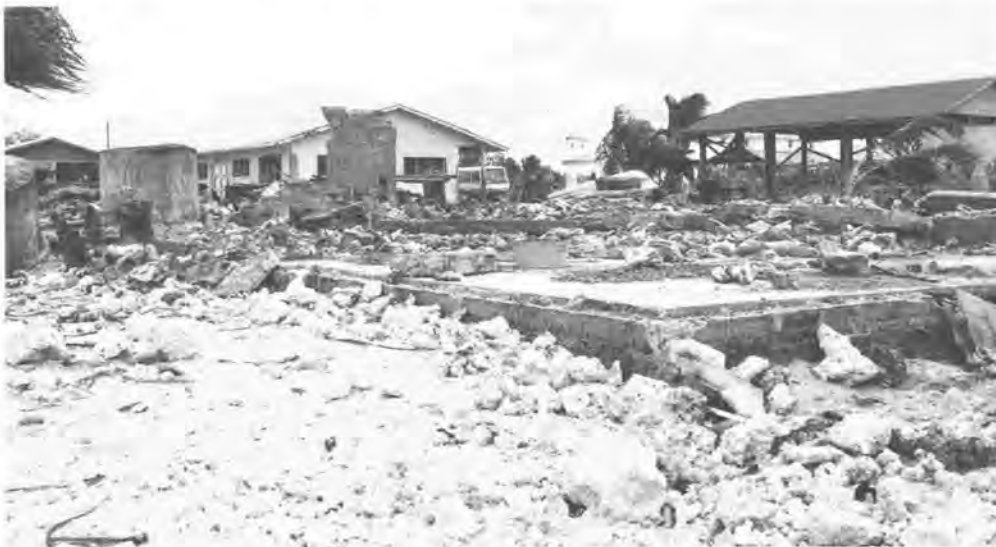
Damage from waves at Vaitupu. (photo: Alefaio Semese)
