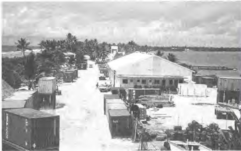
Funafuti wharf is the main storage area for all goods brought into Tuvalu, including chemicals and petroleum products. The wharf is located on a very narrow part of the island, and any liquid spillage will quickly flow into the sea. (photo: Alefaia Semese)
