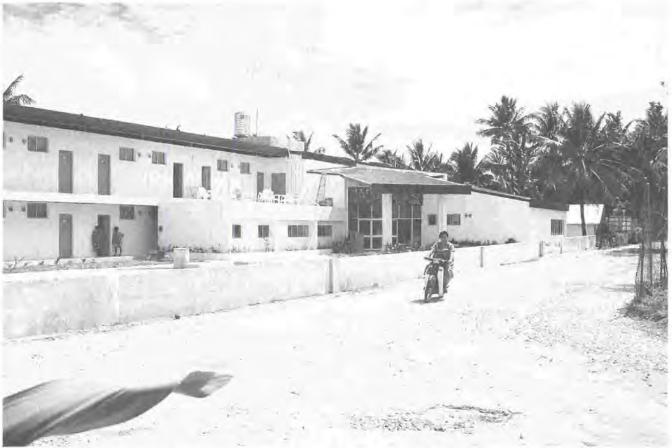
Vaiaku Lagi Hotel. Donor-sponsored development such as this will provide a great economic boost to Tuvalu. However, such developments should be subject to Environmental Impact Assessment (EIA) to ensure they meet agreed environmental standards. (photo: Alefaio Semese)
