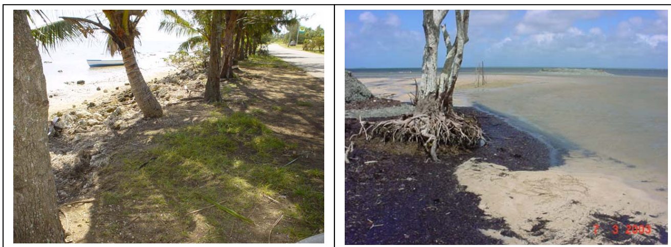
Photo 6: Severe coastal erosion from sand mining
