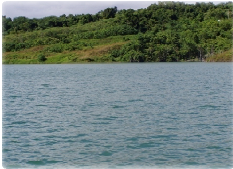
FIG 6.1 Gold Ridge tailings dam Lake – Photo: Ministry of Mines and Energy
