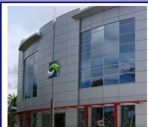
New Samoa Tel headquarters - Providing state of the art technology in ICT essential to the advancement of the private sector.
