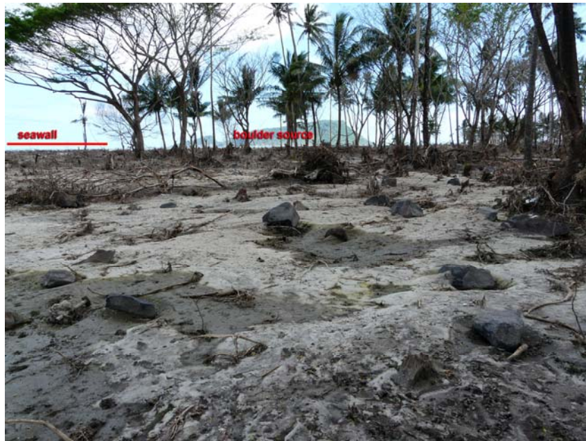
Figure 10: Boulder field and sand sheet at Satitua. In the background, the seawall behaved as a source for boulders
