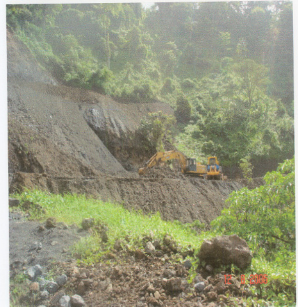
Soils naturally porous, stony and bouldery
