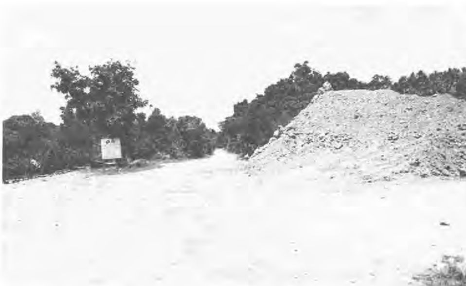
Stockpile of dredged coral materials for road capping at Urung Dock, Ngaraard State. A comprehensive study to assess the overall impact of the current level of dredging in Palau would be valuable. (photo: Demei Otobed)
