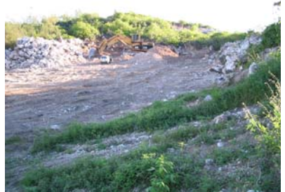
Pit 7, pinnacle removal secondary phosphate mining trial
