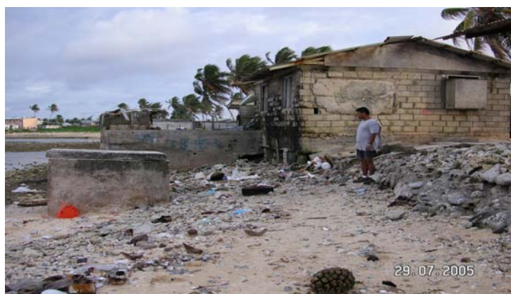
Figure 8: Exposed home on Oceanside of DUD area of Majuro Atoll
