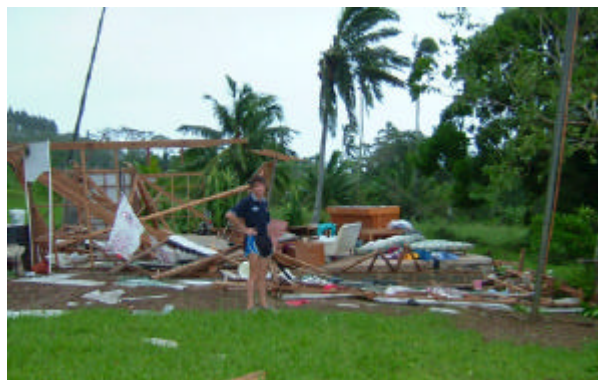
Cyclone damage in Cook Islands
