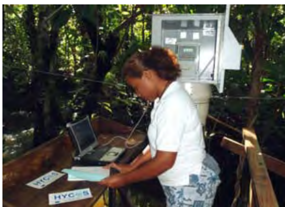
Photograph 7: programming up completed Ngermaskang station
