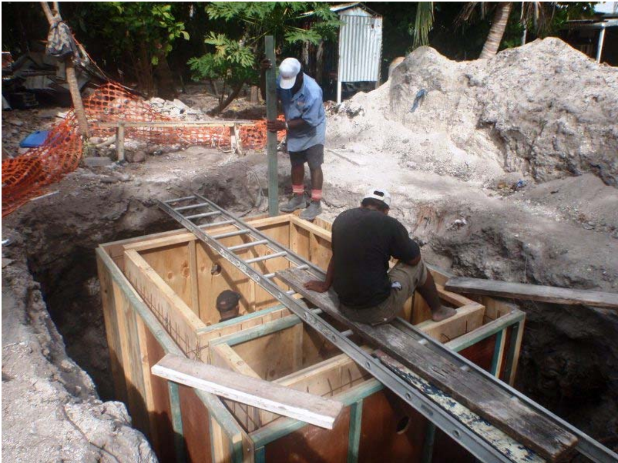
Construction of pilot sanitation systems
