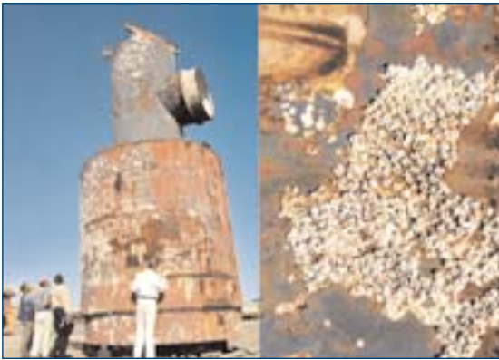
An example of bio-fouling on offshore oil infrastructure
