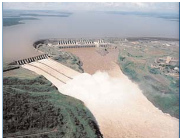
The world's largest hydroelectric plant at Itaipu, already impacted by the Golden Mussel
