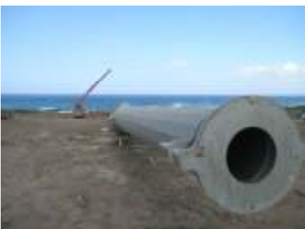
Wind Turbines being erected at the Maddens Wind Farm in Nevis
