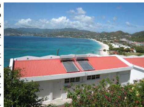
A solar hot water system on a rooftop in St. George's. Systems such as this are a common feature of Grenada's landscape.
