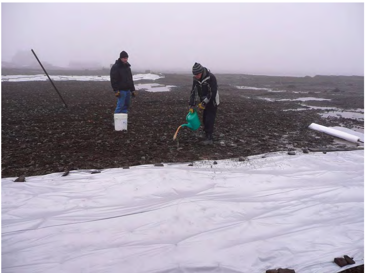
Fig. 6.3.9. Application of 'Devouroil' biological product
