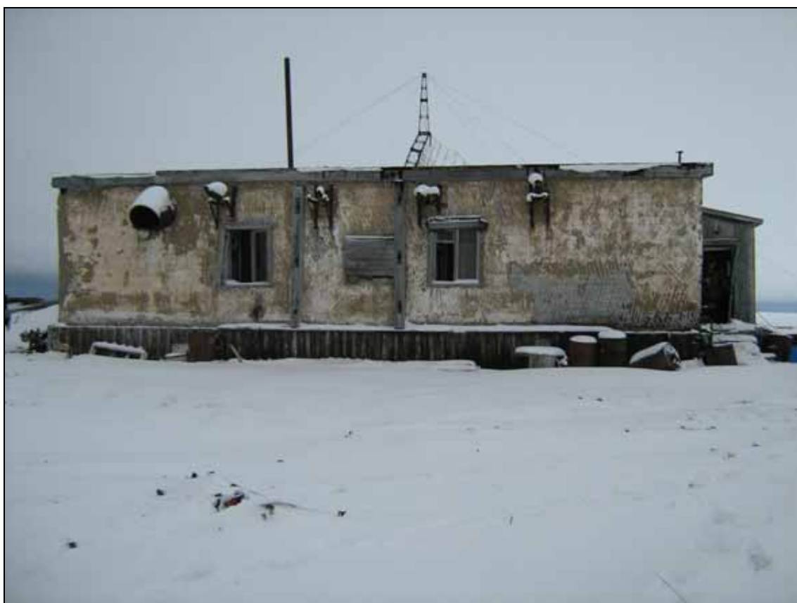
Photo 5.2 Diesel plant building
