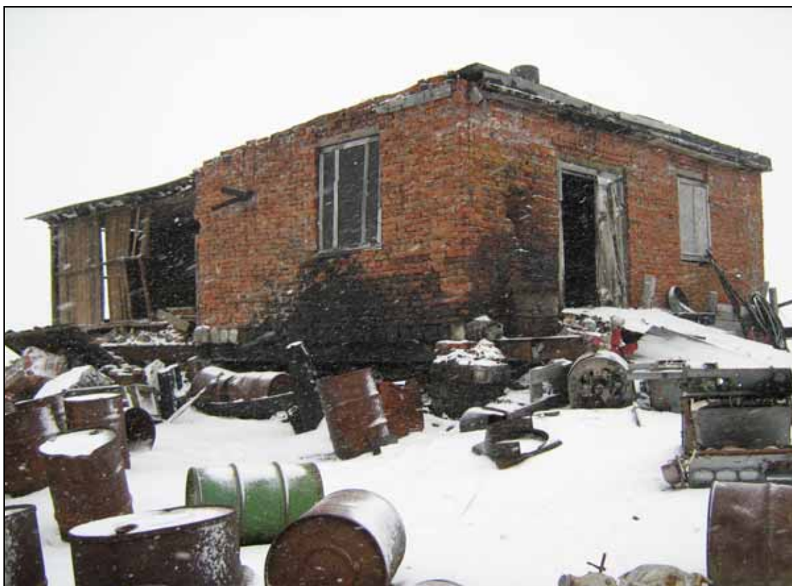
Photo 4.13 Destroyed Diesel plant building
