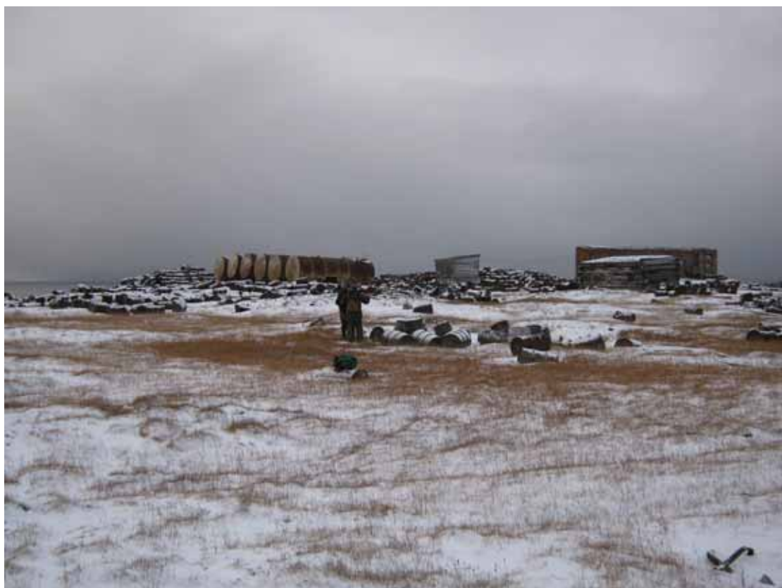
Photo 4.7 Cisterns near the Diesel plant
