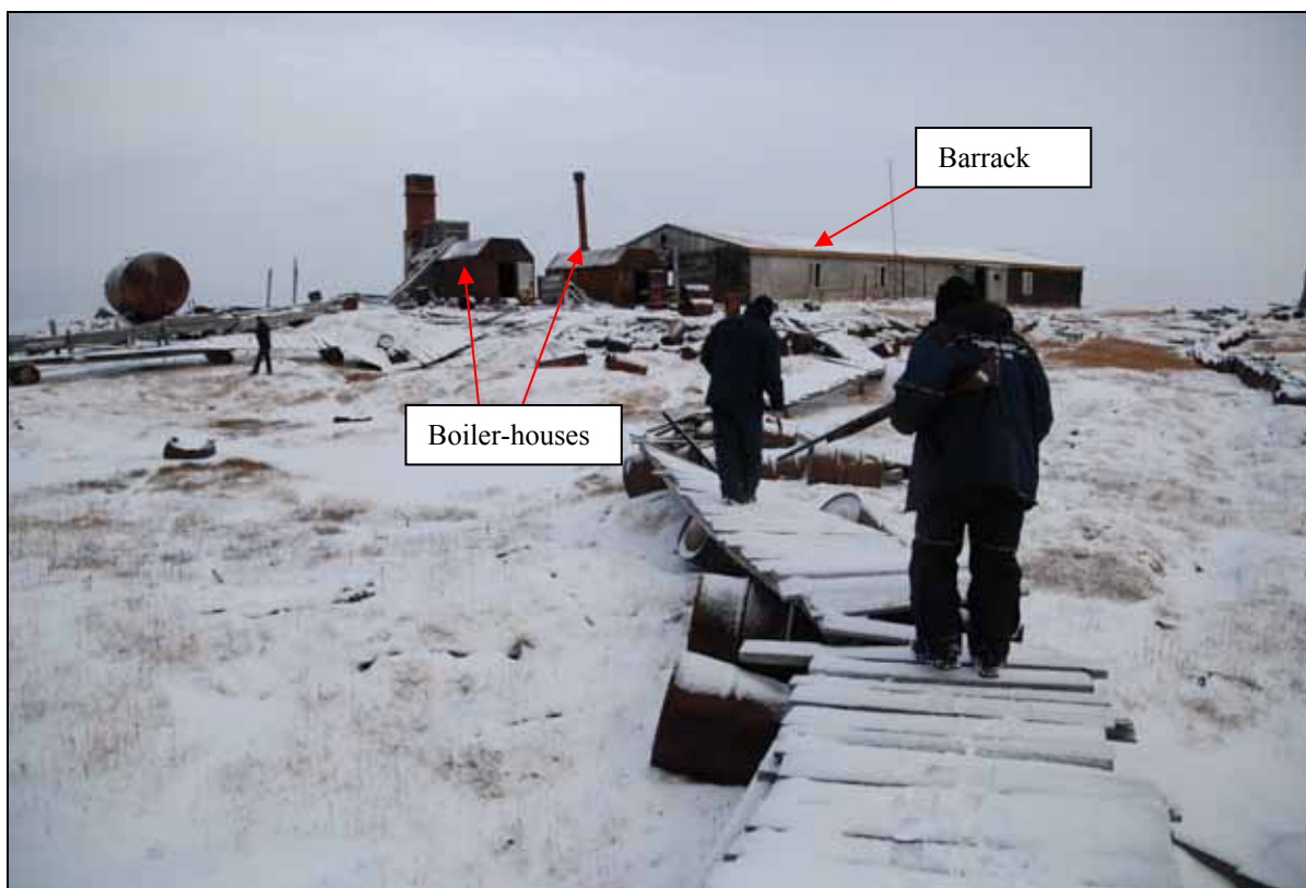
Photo 4.19 Boiler-house and Diesel plant near the barrack
