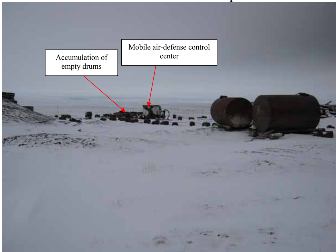
Photo 5.13 View of empty cisterns from north-east part
