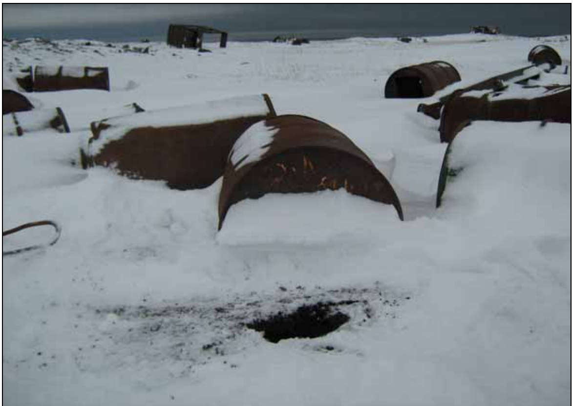
Photo 5.9 Leak of fuel and lubricants on the west side of the Diesel plant building
