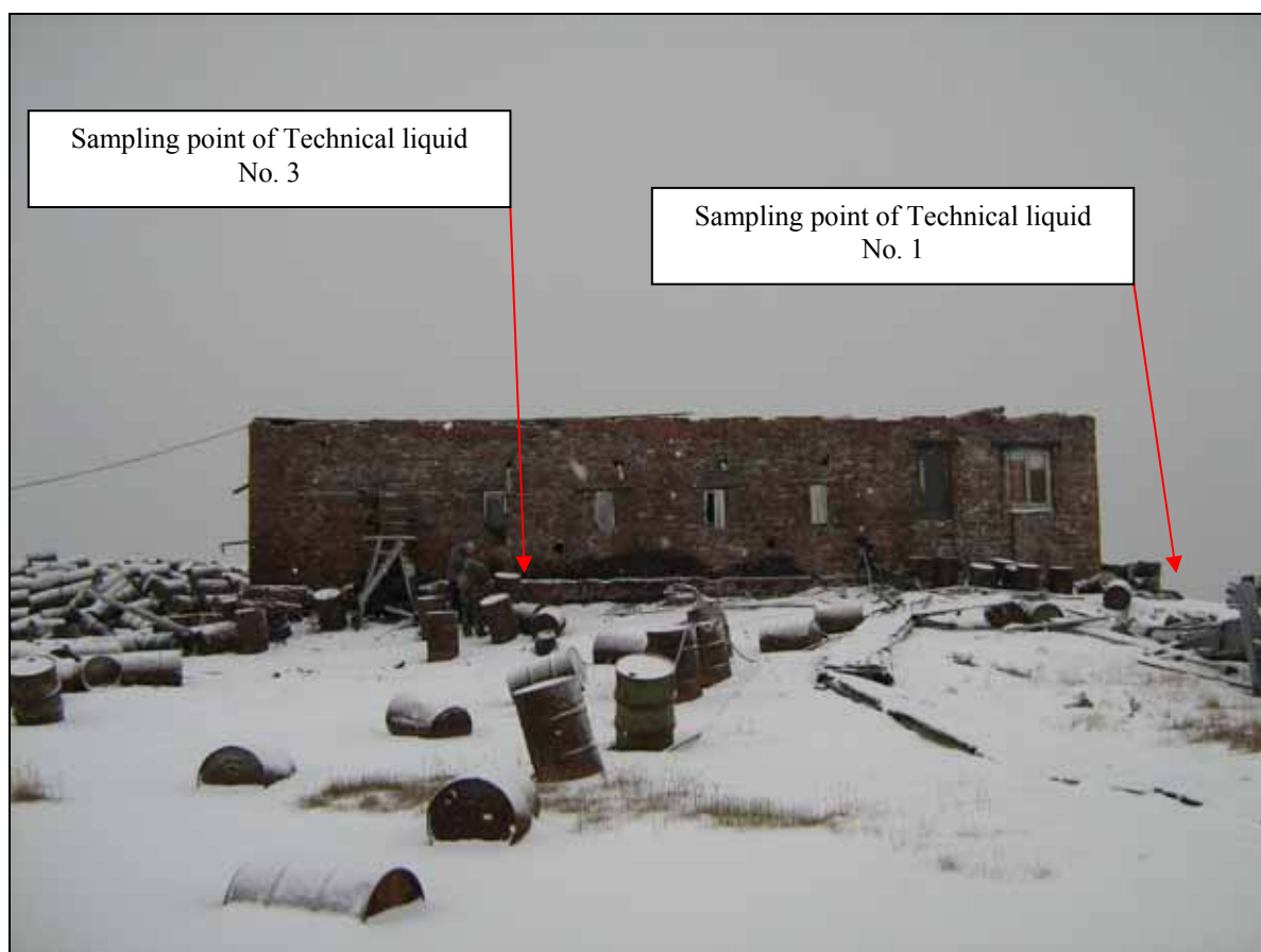
Photo 4.5 View of the Diesel plant building from the north side
