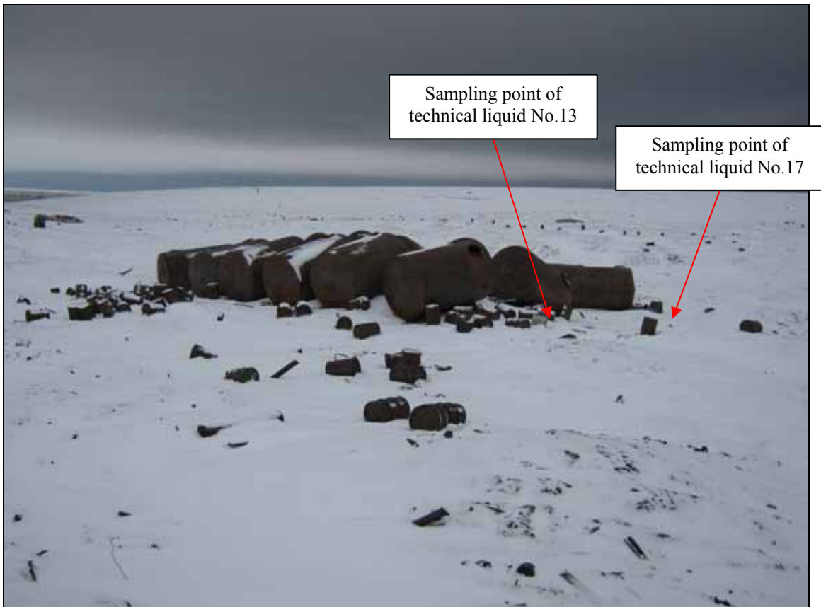
Photo 5.20 Empty cisterns and drums scattered around them, located on the left bank of no-name creek No.4
