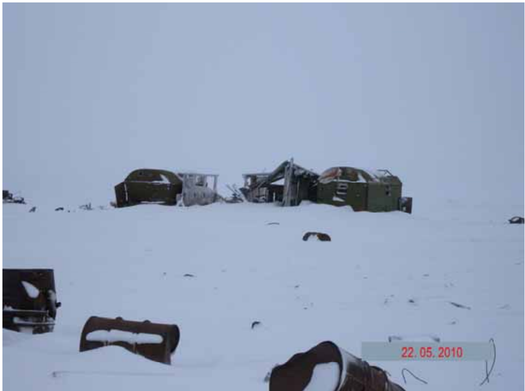
Picture 2.2.26 Destroyed building of the radar station commandant's office observation
