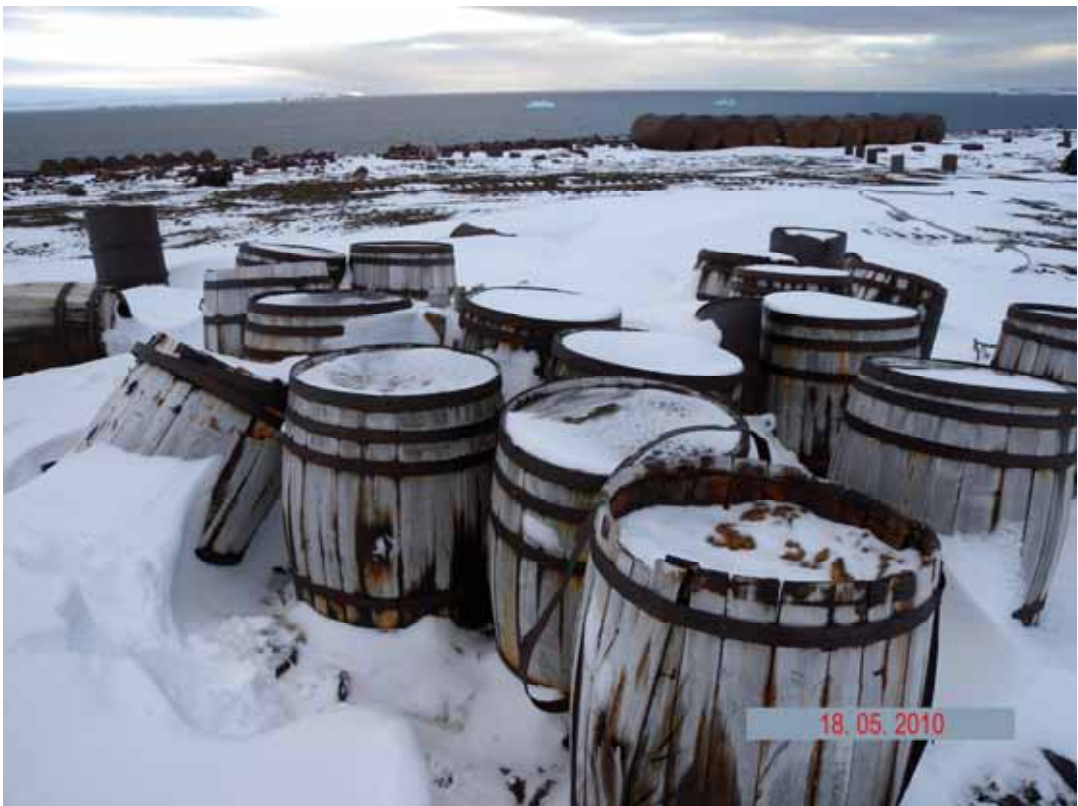
Picture 2.2.12 Accumulation of wooden drums with semisolid lubricant in the surveyed area of fuel and lubricant storage facility near the Severnaya Bay
