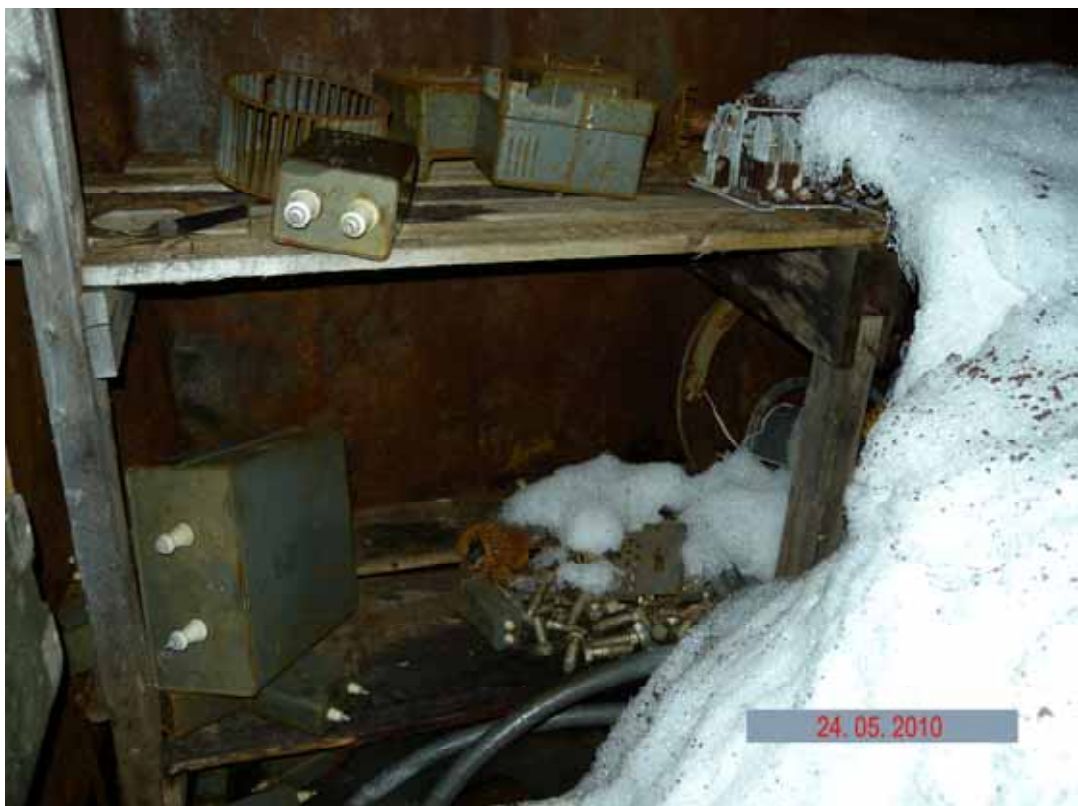
Picture 2.2.32 PCB-containing inside the condenser and transformer storage facility in the surveyed area of the radar station
