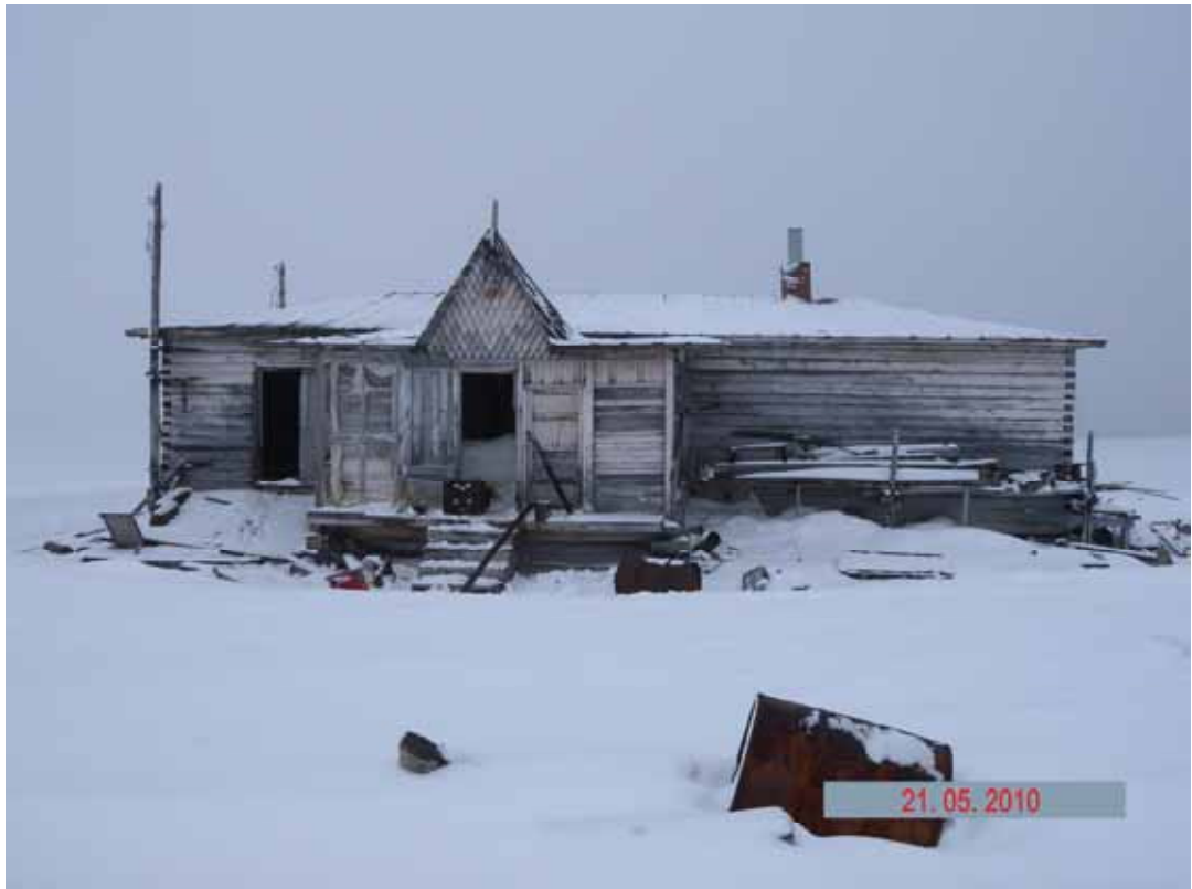
Picture 2.2.19 Diesel building (site 280) in the territory of the abandoned polar station
