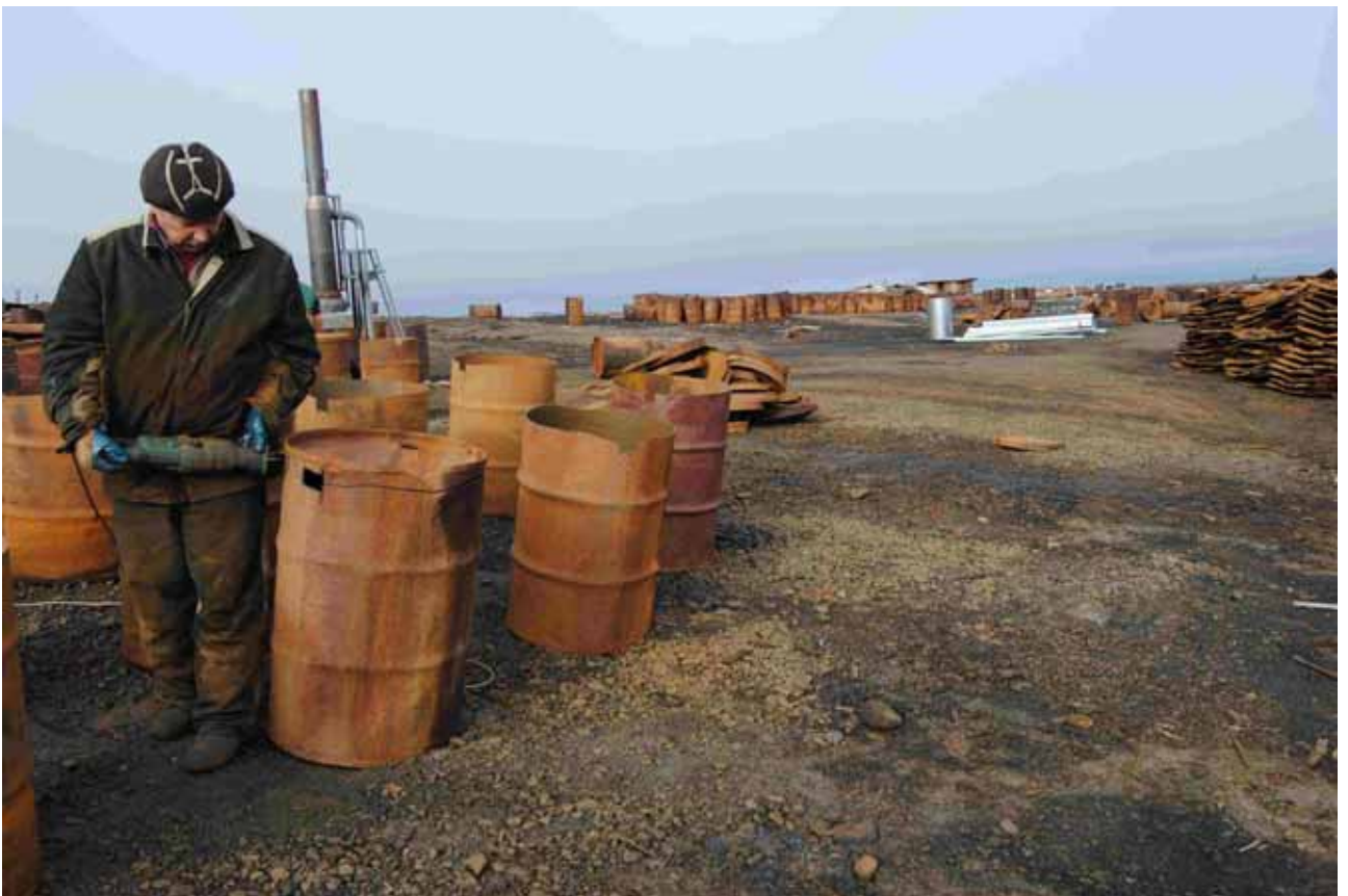
Figure 14.6. Drum broaching using reciprocating saw
