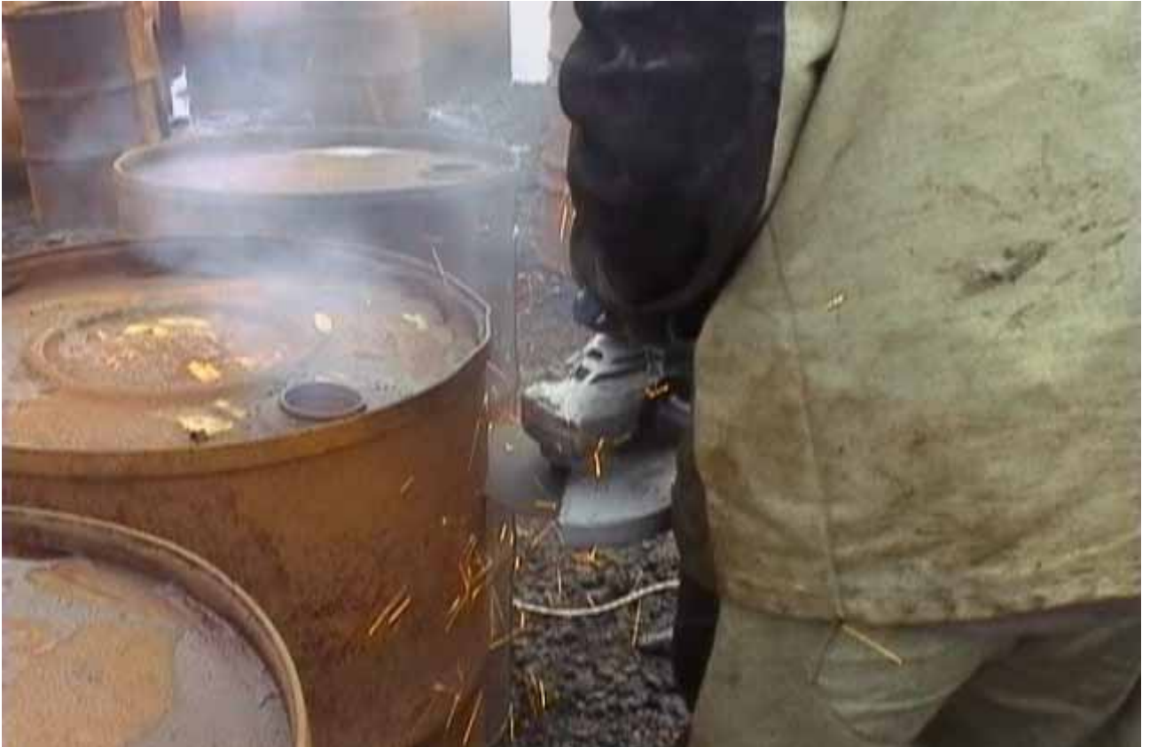
Figure 14.7. Drum breaching using angle grinder
