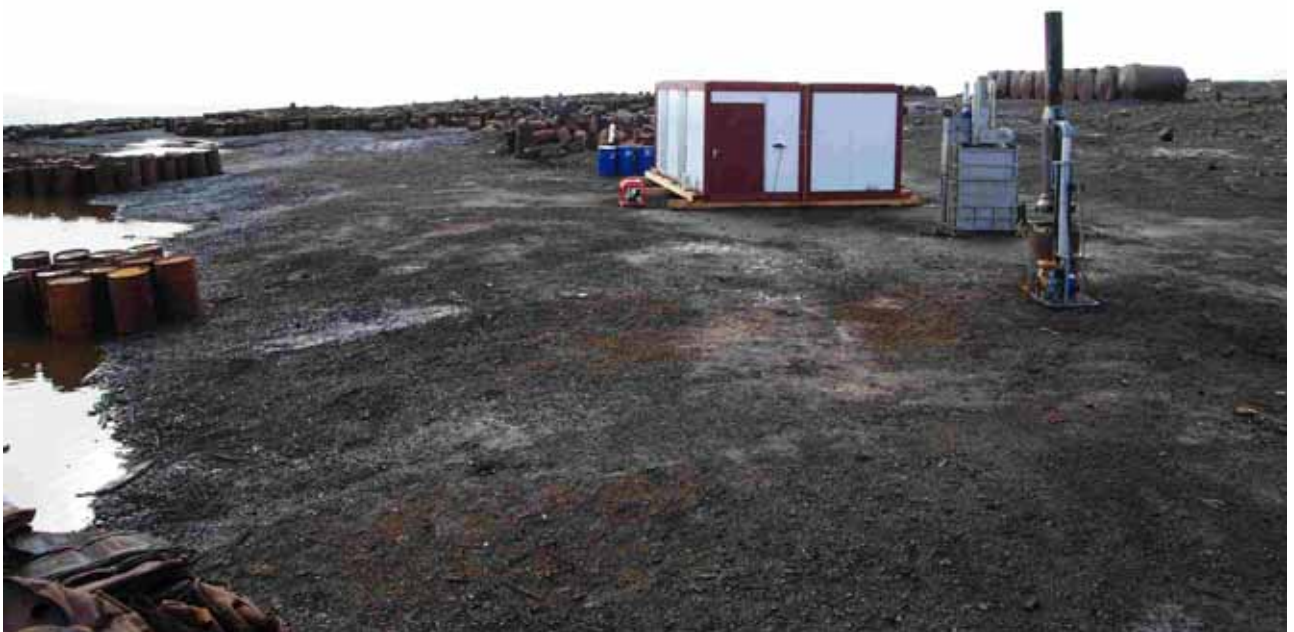
Figure 13.4. General view of job site
