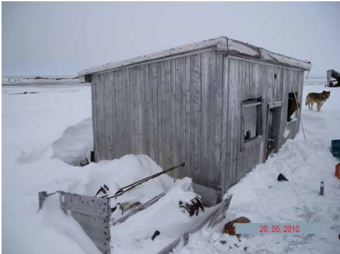
Picture 2.2.29 Condenser and transformer storage facility (site 164) in the surveyed area of the radar station
