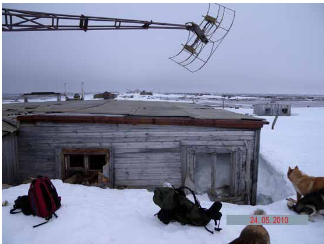
Picture 2.2.34 Antenna and radar station building (items No. 169, 170) in the surveyed area of the radar station
