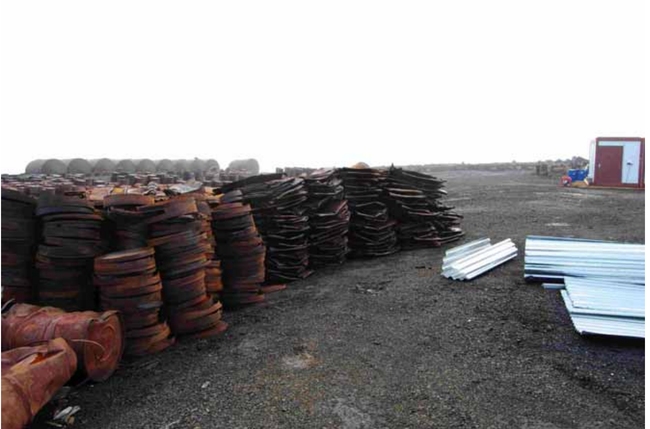
Figure 14.12. Compacted drums prepared for loading.
