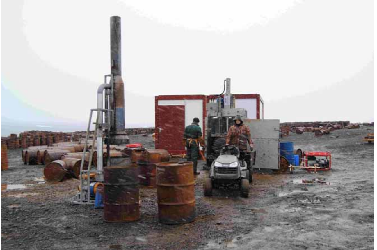
Figure 14.5. Progress of work on the site. In the foreground – minitractor CRAFTSMAN 28908
