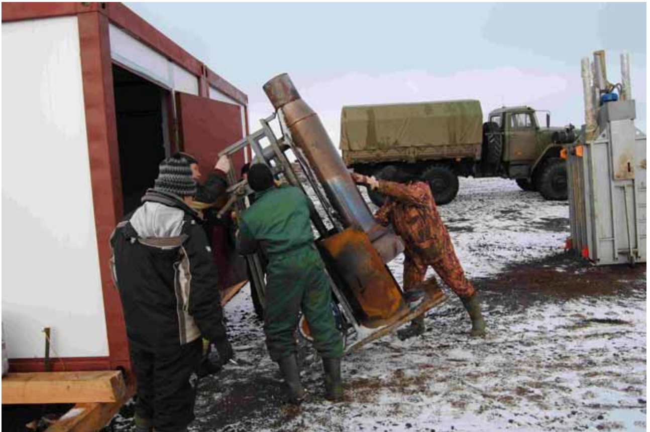
Figure 13.7. Installation of “Fakel -1M”;
