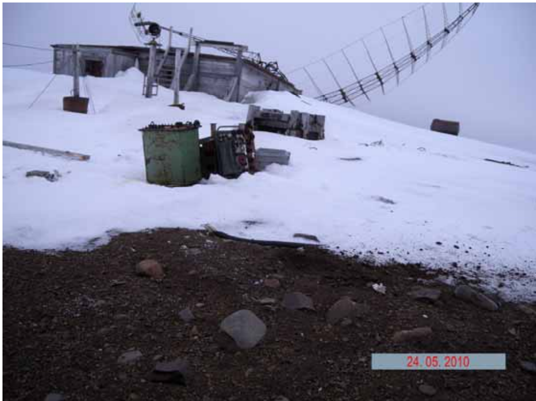
Picture 2.2.35 Transformers, Antenna and radar station building (items No. 142, 145), in the surveyed area of the radar station
