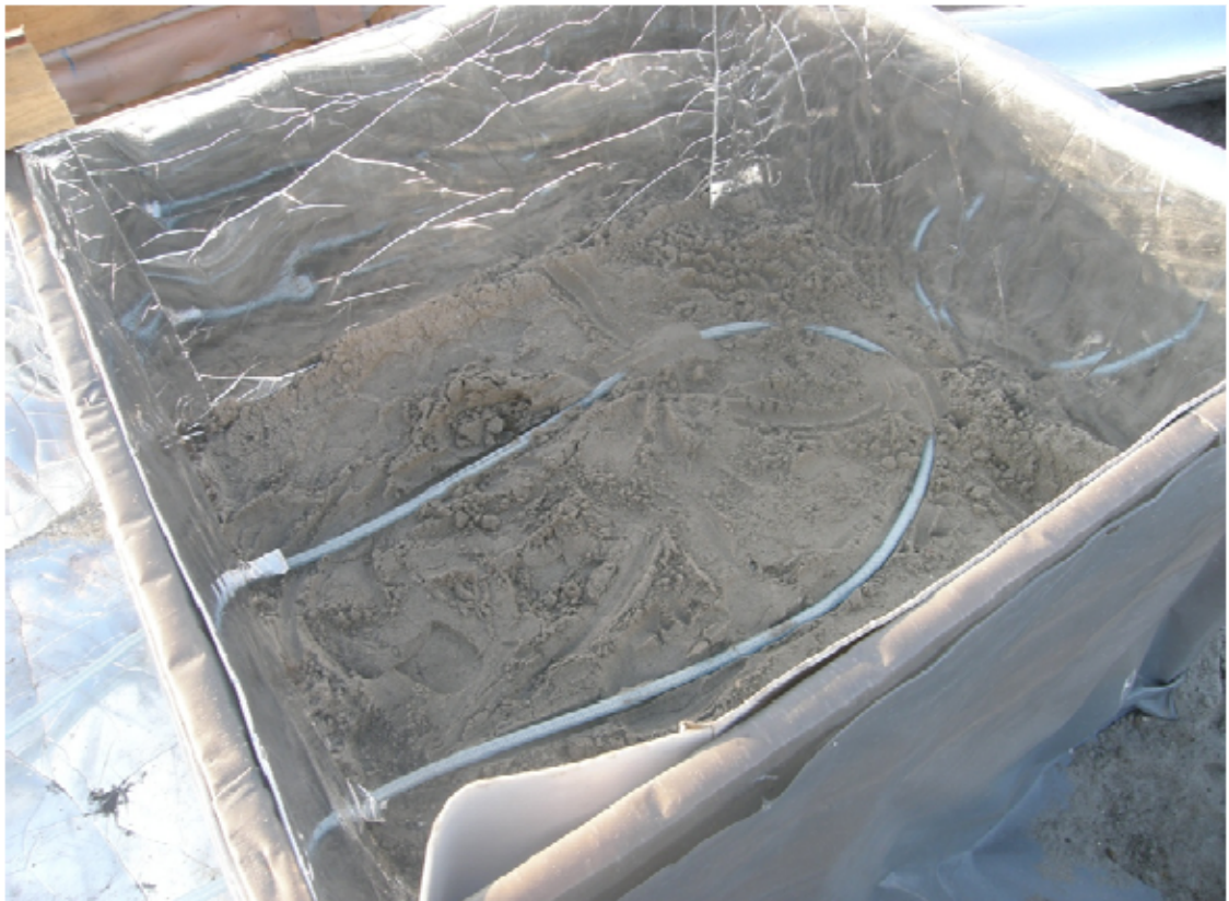
Picture 5d organisation System thermal insulator and dewaterings of meshes in an engineering part of range with stacking of a net of perforated pipes for soil aeration
