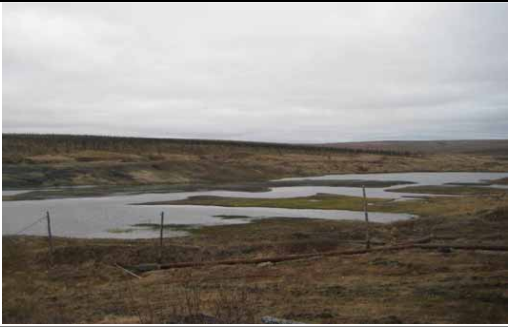
Photo 4 Intermediate dam built of peaty ground
