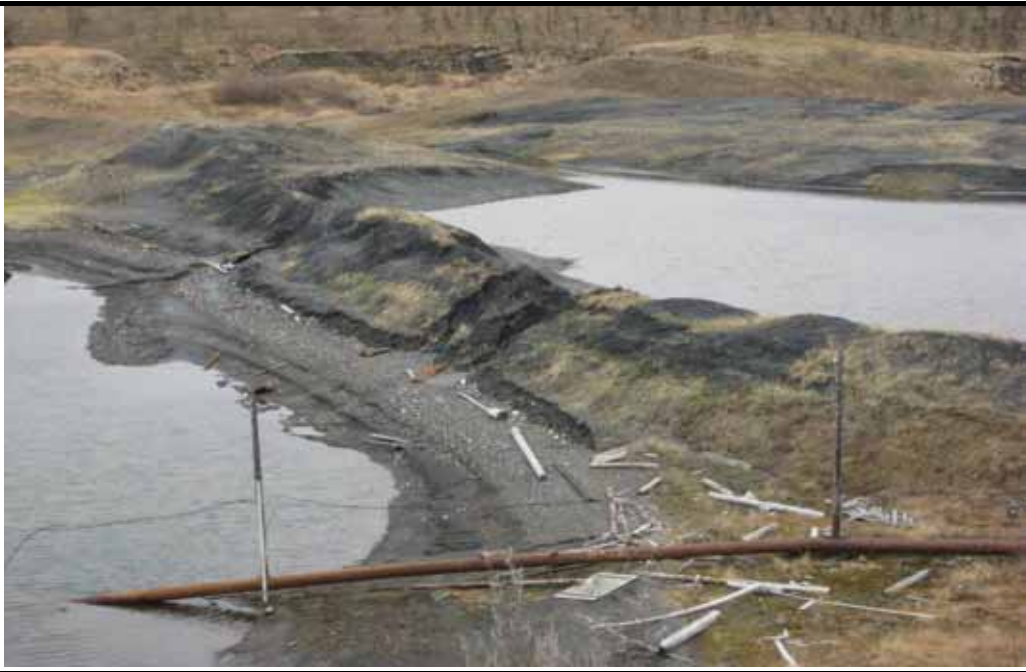
Photo 4 Intermediate dam built of peaty ground
