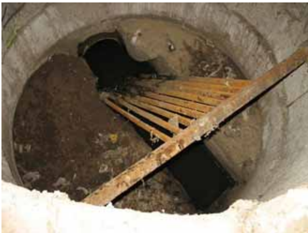
Photo 3. Screen for retention of large debris
