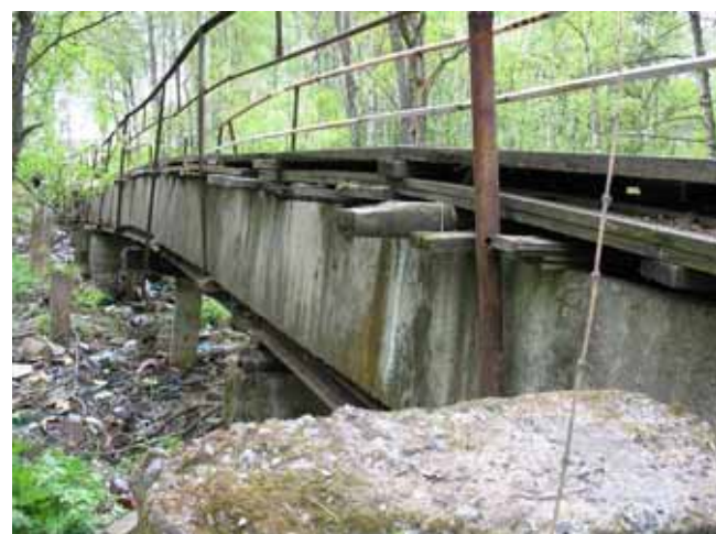
Photo 10. Overpass at the sewage network
