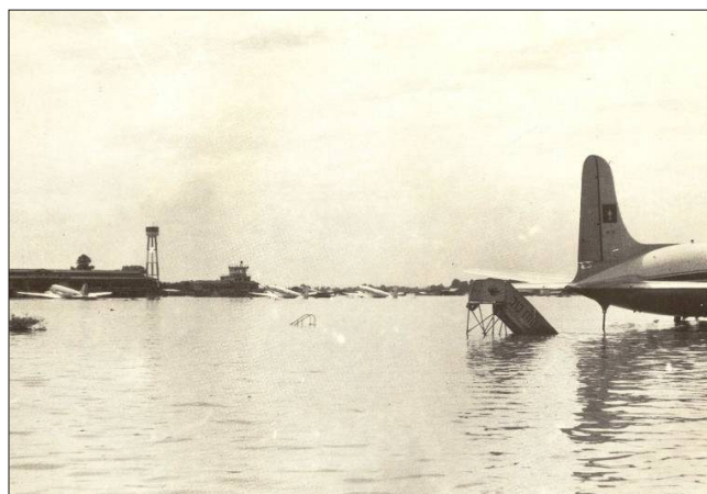
The flooded runway at Wattay Airport.
