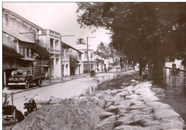
Sandbags were laid to protect the river banks.
